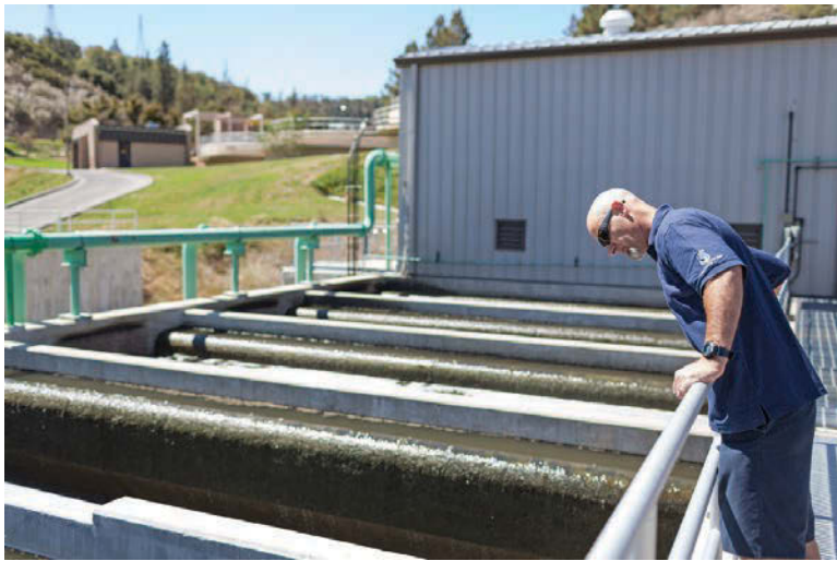
Trevor Cory visually checks the plant's denitrification filter bed (Severn Trent).
