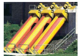
Screw pump restoration from Evoqua Water Technologies
