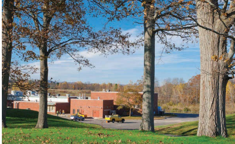
Pittsfield combined heat and power building. (Photos by David Lamb Photography)
