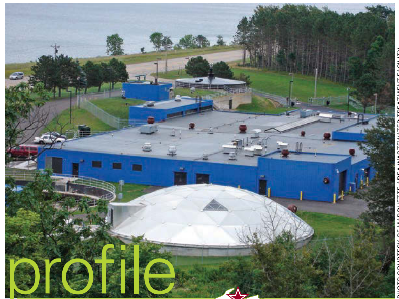
PHOTO COURTESY OF MARQUETTE AREA WASTEWATER TREATMENT FACILITY
