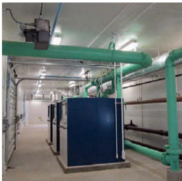
Blowers and piping for three digesters are assisted by dissolved oxygen monitoring to optimize aeration and energy usage.
