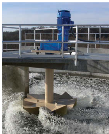
The impeller's design on a low-speed LANDY-7 surface aerator (WesTech Engineering) increases oxygen transfer efficiency and reduces axial and radial loads.
