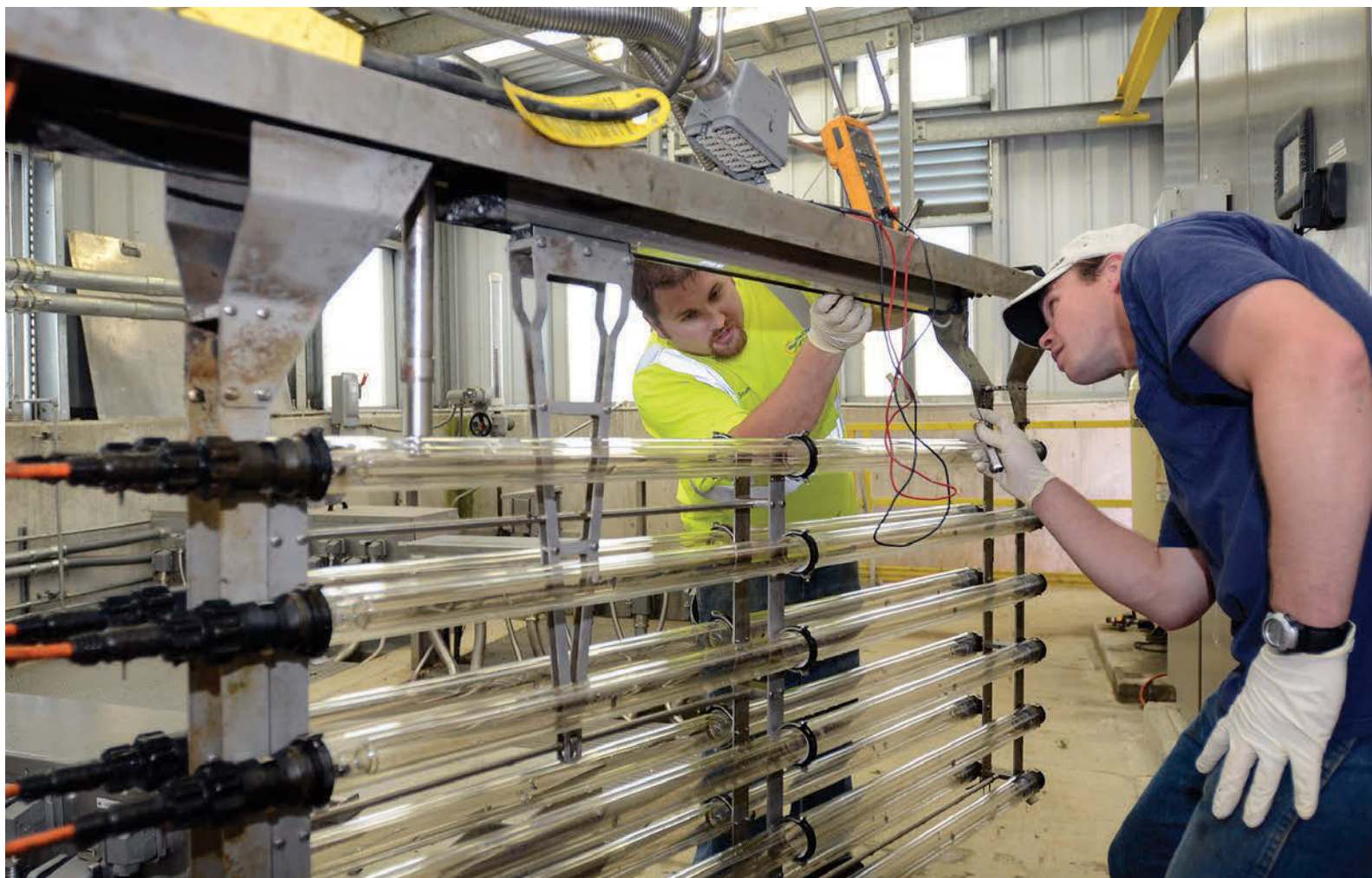
ABOVE: Operators Scott Yonkers (left) and Bill Poelma replace modules in the plant's UV disinfection system. LEFT: The Grandville plant has seen substantial upgrades since 2006.
