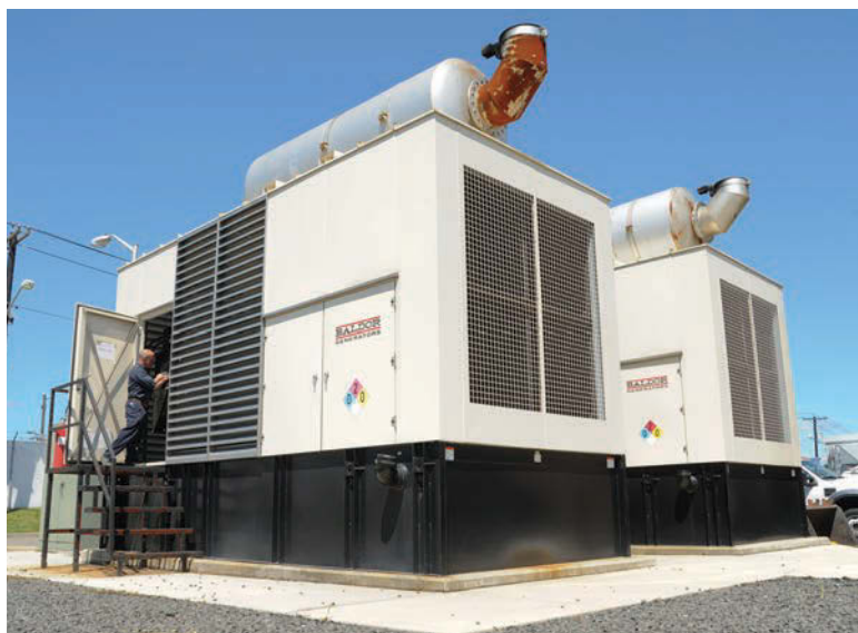
The plant has two diesel-fueled engines (Mitsubishi) with Baldor (Generac) generators. Rob Remite, electrician, is shown performing maintenance.
