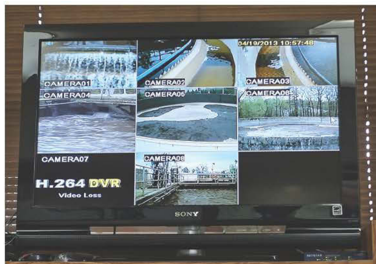
A closed-circuit TV system helps the plant staff monitor the facilities.
