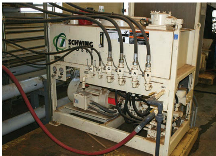
The power pack for the plant's Schwing sludge pumps.
