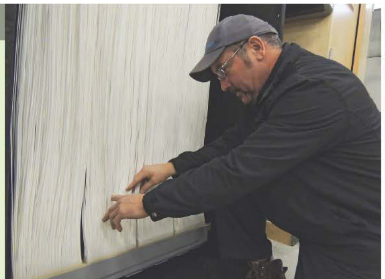
Mark Yasinski inspects the demonstration model of the GE Zeeweed 500D hollow-fiber membrane modules in the bioreactor.
