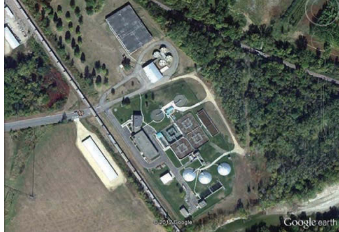
Aerial view of the New Ulm Wastewater Treatment Plant.
