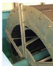
Bio-Wheel fixed-film aerator from H2O Innovation
