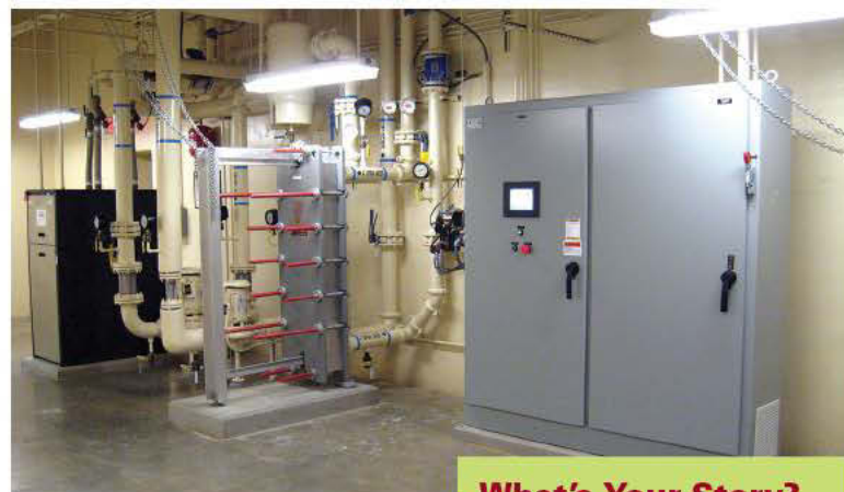
The heat pump and the control system for the final clarifier.
