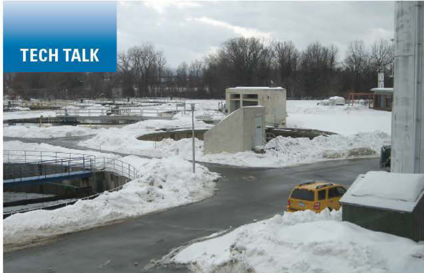
Two of three 70-foot-diameter primary clarifiers (WesTech) are visible on the right, one of three 82-foot-diameter secondary clarifiers is on the left, and the three aeration tanks (624,000 gallons each) are in the background.
