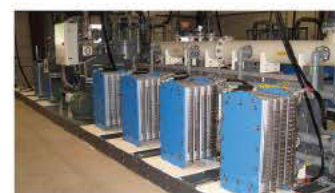
Klorigen chlorine and sodium hypochlorite plant from Electrolytic Technologies Corp.
