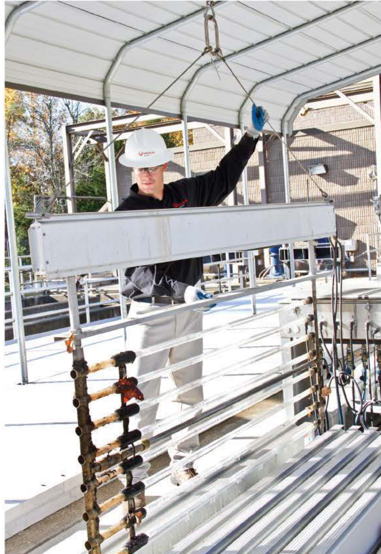
Justin Metz conducts a preventive maintenance inspection on a UV module from the TrojanUV3000Plus system.
