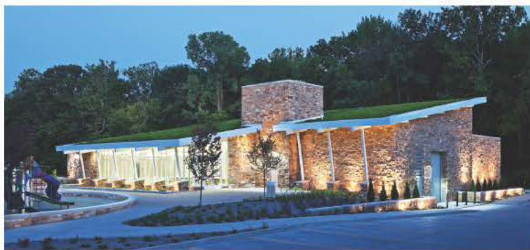
A sloped green roof planted with sedum, green mantle and dragon's blood covers the community room, which has space for 50 people.
