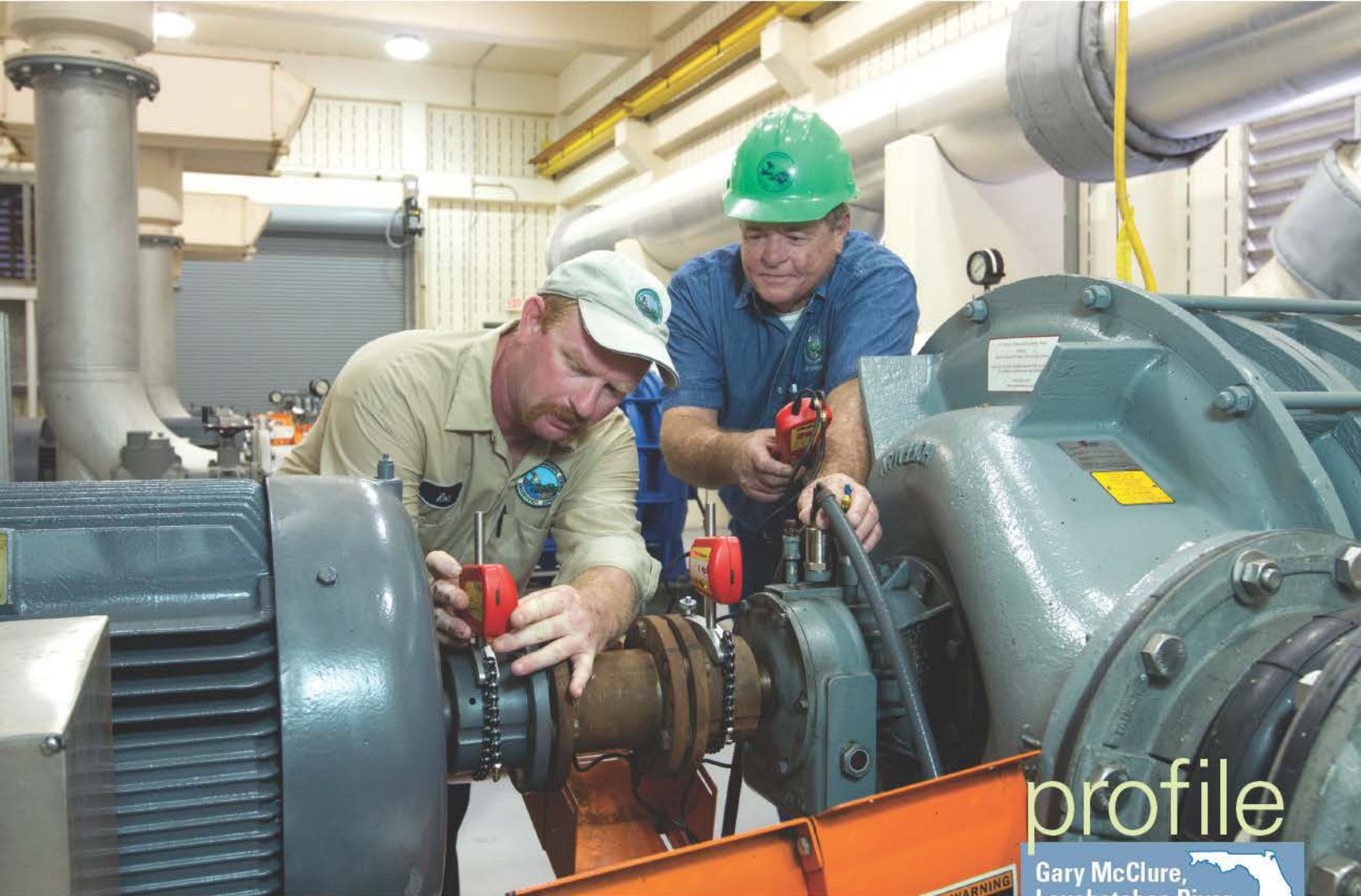
ABOVE: Operator Ron King, left, and Gary McClure use a laser alignment tool (VibrAlign) to align the main blower drive coupling (Hoffman and Lamson, Gardner Denver Products). Alignment on high-speed blowers helps ensure long bearing life and efficient operation. BELOW: The Loxahatchee River Environmental Control District provides irrigation-quality water to surrounding golf courses. The Busch Wildlife Sanctuary is located on site.
