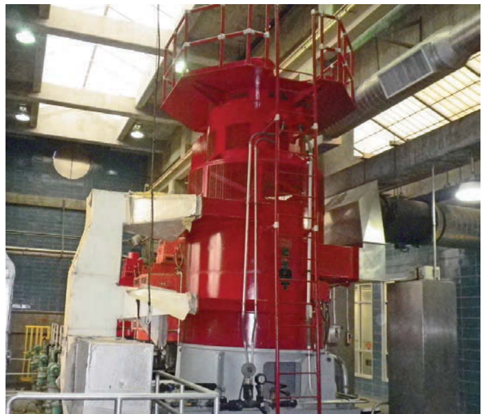
The clutch and motor atop the 1,650 hp Peerless pump make the unit three-stories high.
