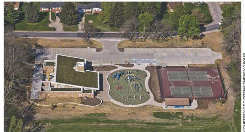
The newly renovated Juan Solomon City Park is built atop a 38 mgd lift station that helps deliver wastewater to the city's Belmont Advanced Wastewater Treatment Facility.
