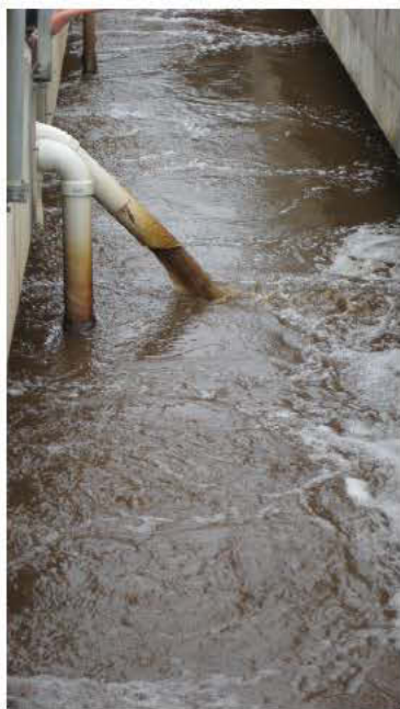
A NovaThermal unit extracts thermal energy from wastewater in a mixed liquor channel to fulfill the heating needs of the plant's compressor building and gallery.
