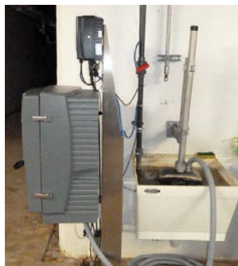
LEFT: Rob Minnema, utility foreman, checks the parameters on the sc1000 digital controller, part of the Hach phosphorus control system. BELOW: The system includes a PHOSPHAX sc phosphate analyzer (left), sc1000 digital controller (above), and Filtrax probe in a sample tub.
