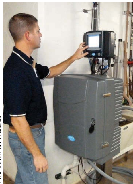
LEFT: Rob Minnema, utility foreman, checks the parameters on the sc1000 digital controller, part of the Hach phosphorus control system. BELOW: The system includes a PHOSPHAX sc phosphate analyzer (left), sc1000 digital controller (above), and Filtrax probe in a sample tub.
