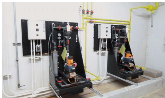
The ProMinent ferric chloride pump system at the Beaver Dam Wastewater Treatment Plant.
