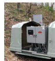
StationComm automated alarm system from Smith & Loveless
