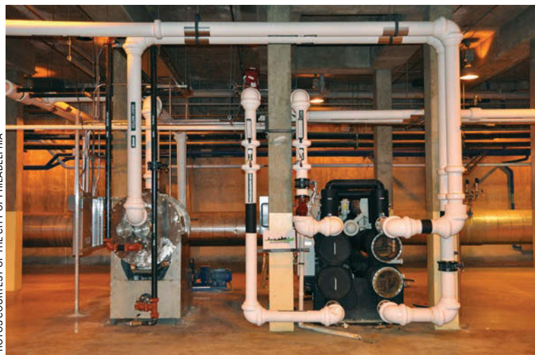
The geothermal installation consists of a heat pump, filter and the piping needed to extract thermal energy from the wastewater.
