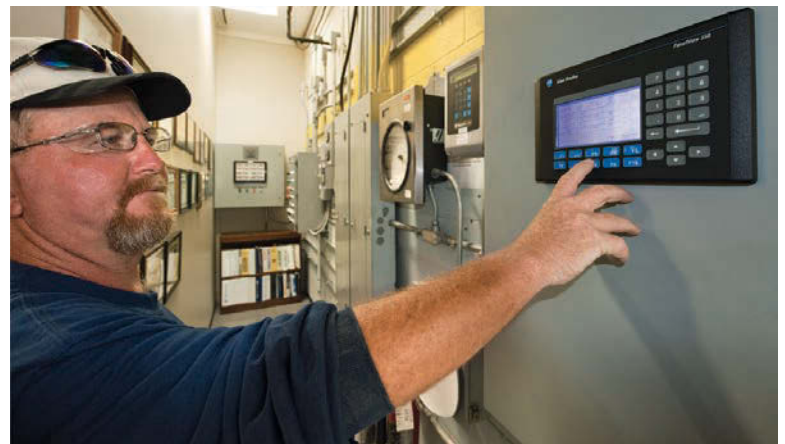
Ken Riley checks the programmable logic controller (Allen-Bradley/Rockwell Automation) that controls activated sludge return rates from the clarifier.
