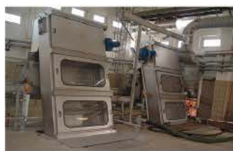
FSM/WasteTech multi-rake bar screens from Kusters Water
