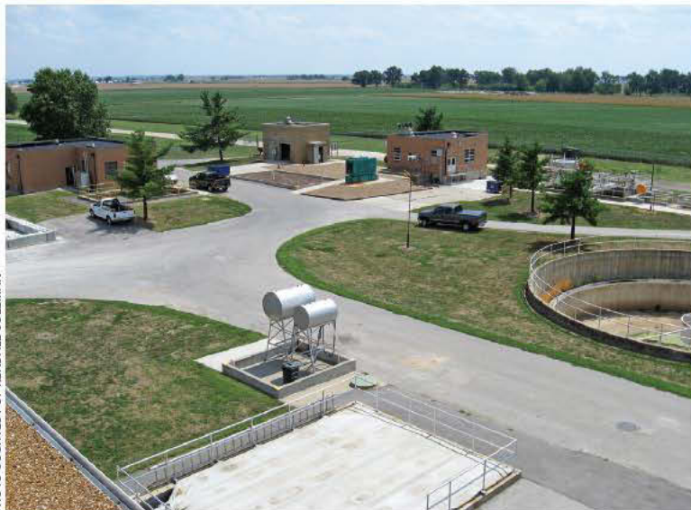
The Mississippi River plant (7.5 mgd design) is operated by the American Water Contract Services Group, through Environmental Management Corp.
