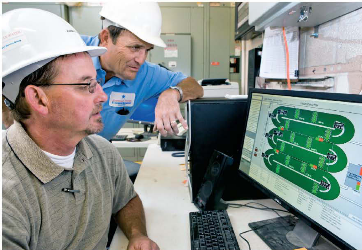
Operator Robert Lippincott, right, and facilities manager Kendall Coleman check a secondary treatment process via the SCADA system at the operations control center.
