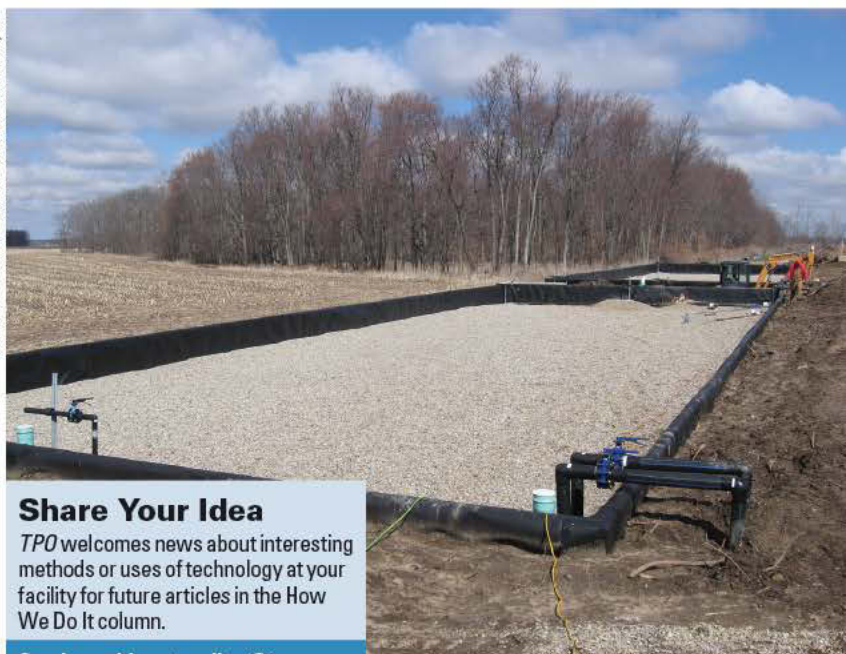
The SAGR system at the Mentone Wastewater Treatment Plant.
