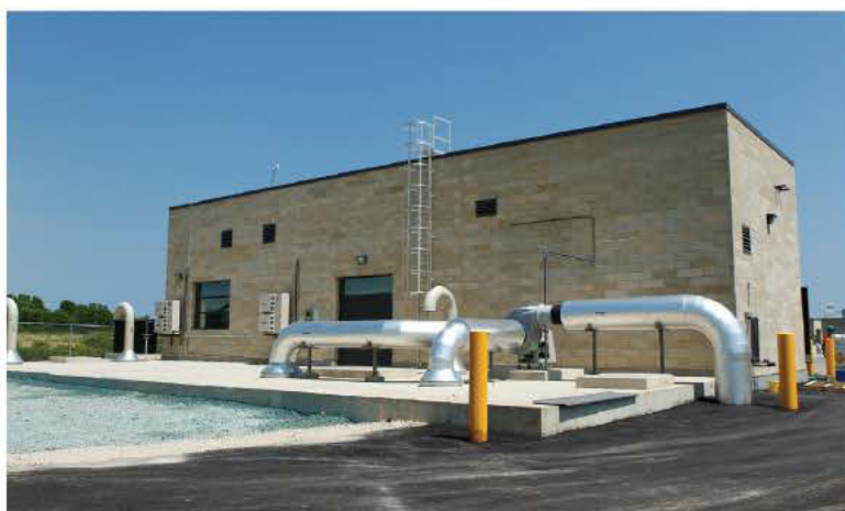
The aerobic digester at the northwest side of the administration building is fitted with an odor-control system.
