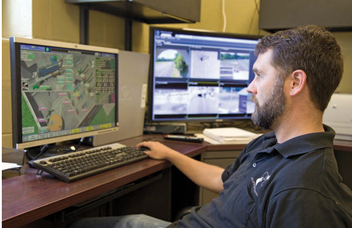
Chief wastewater plant operator Brandon Traugher checks plant operations on the SCADA system from a central office.
