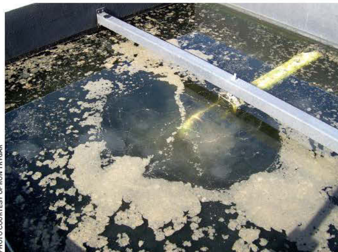
Cooking oil enters a clarifier and rises to the surface.
