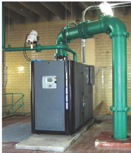
Turblex blowers have improved aeration at the Wausau Wastewater Treatment Plant while also reducing energy needs.
