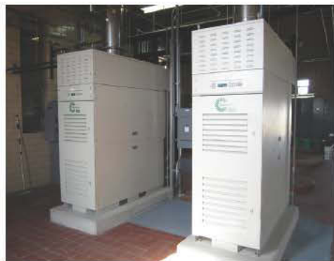
Two Capstone 65 kW microturbines will help the plant avoid buying nearly 1 million kWh and 77,000 therms of natural gas from the local utility every year.
