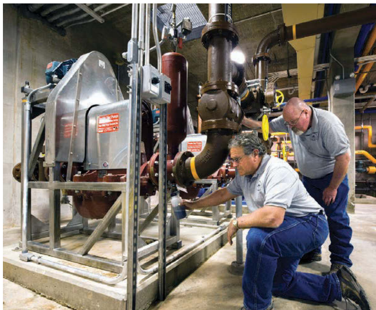
Plant maintenance manager Bob Jones, left, and biosolids lead worker Ron Lacina take a sample from one of two new Double Disc pumps (Penn Valley Pump).
