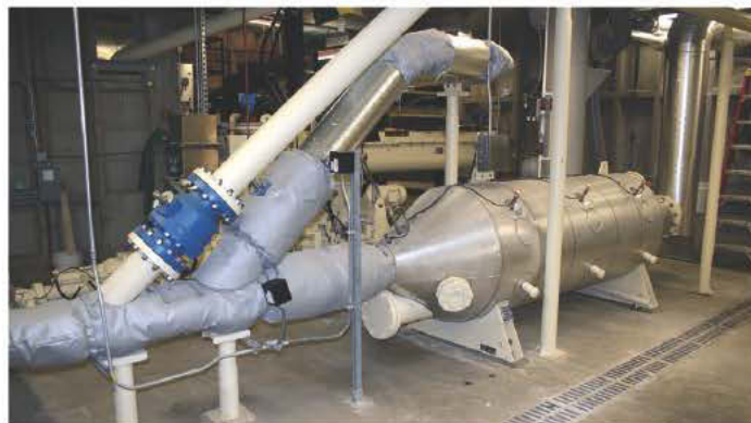
In the insulated Bioset reactor, biosolids are kept at a constant 158 degrees F for at least 30 minutes to ensure that all pathogens are neutralized.
