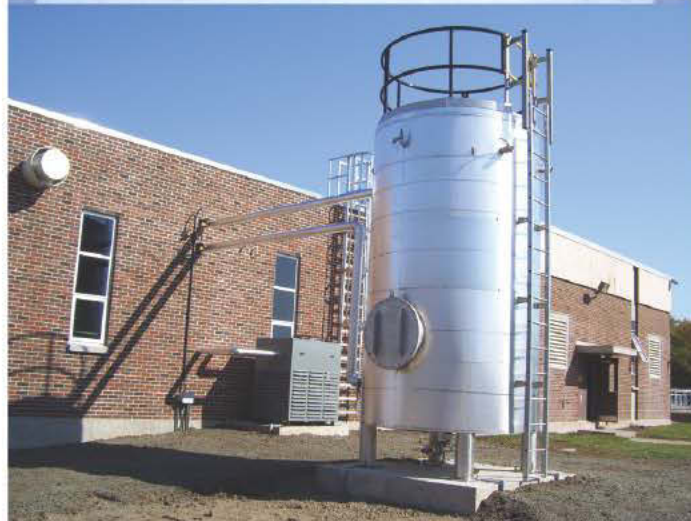
The gas treatment skid (Unison) removes contaminants like organic siloxanes from the biogas to protect the microturbines. The hydrogen sulfide removal vessel is located outdoors next to the plant.
