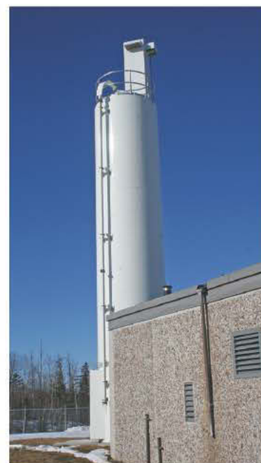
Lime for the Bioset process is stored in a 1,560-cubic-foot silo next to the storage pad.
