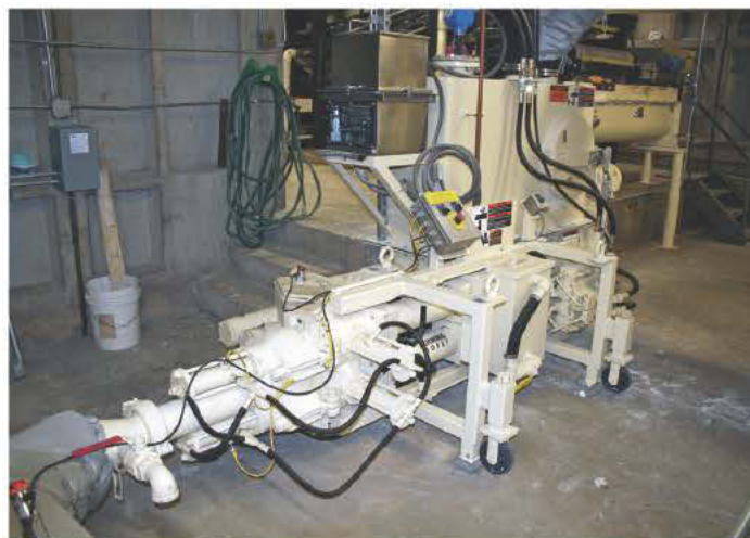
Treated biosolids are pumped under pressure by a Schwing KSP-5 piston pump to an insulated reactor. The sulfamic acid feeder (stainless steel container) is mounted atop the pump.
