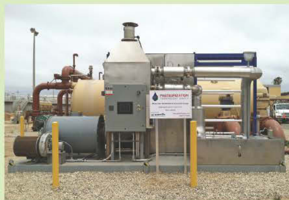
X-500 wastewater treatment system from the Pasteurization Technology Group (PTG)
