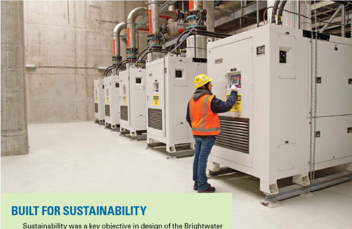
ABOVE: Pumps for membrane bioreactor backflushing (Fairbanks Morse). LEFT: Operator Pam Restovic monitors high-efficiency turbo blowers (APG-Neuros).
