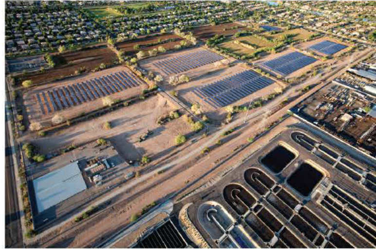
The photovoltaic array at the Neely wastewater plant uses a single-axis tracking system to follow the sun across the sky, increasing output by about 20 percent over a non-tracking installation. When the groundwater recharging basins are filled with water, the panels will provide shade to reduce evaporation losses.
