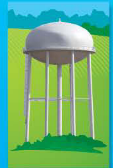
Tank and Well Control
