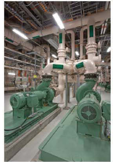
ABOVE: Pumps for membrane bioreactor backflushing (Fairbanks Morse). LEFT: Operator Pam Restovic monitors high-efficiency turbo blowers (APG-Neuros).
