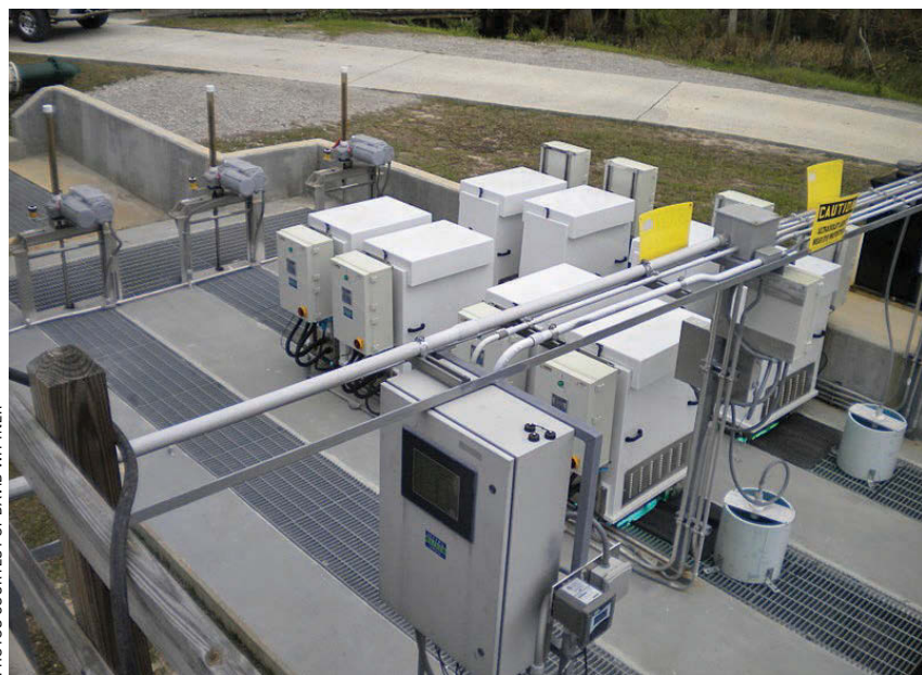
The Mandeville plant has eight OCS 660 microwave UV modules with 16 bulbs each installed in two trains of four. The third channel is for future expansion.
