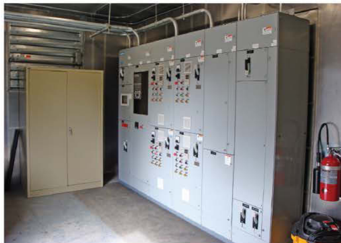
The variable-speed drives on four Flygt pumps are run from this motor control center. Improved energy efficiency will save nearly $70,000 a year.
