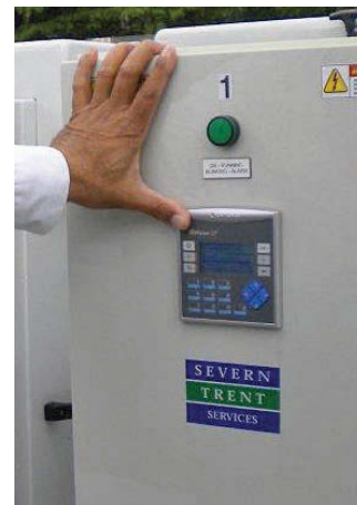
Henry Evans, assistant superintendent at the Mandeville Wastewater Treatment Plant, uses the touch screen to program a MicroDynamics microwave UV disinfection module from Severn Trent Services.
