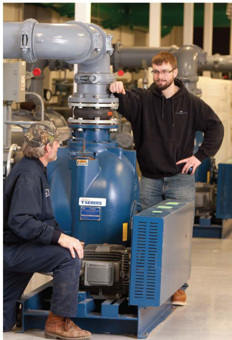
Public Works employee Marty Keyser, left, and Jared Driscoll work on a permeate pump (Gorman-Rupp).
