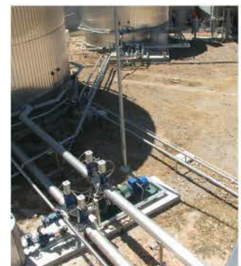
Digester Recirculation
