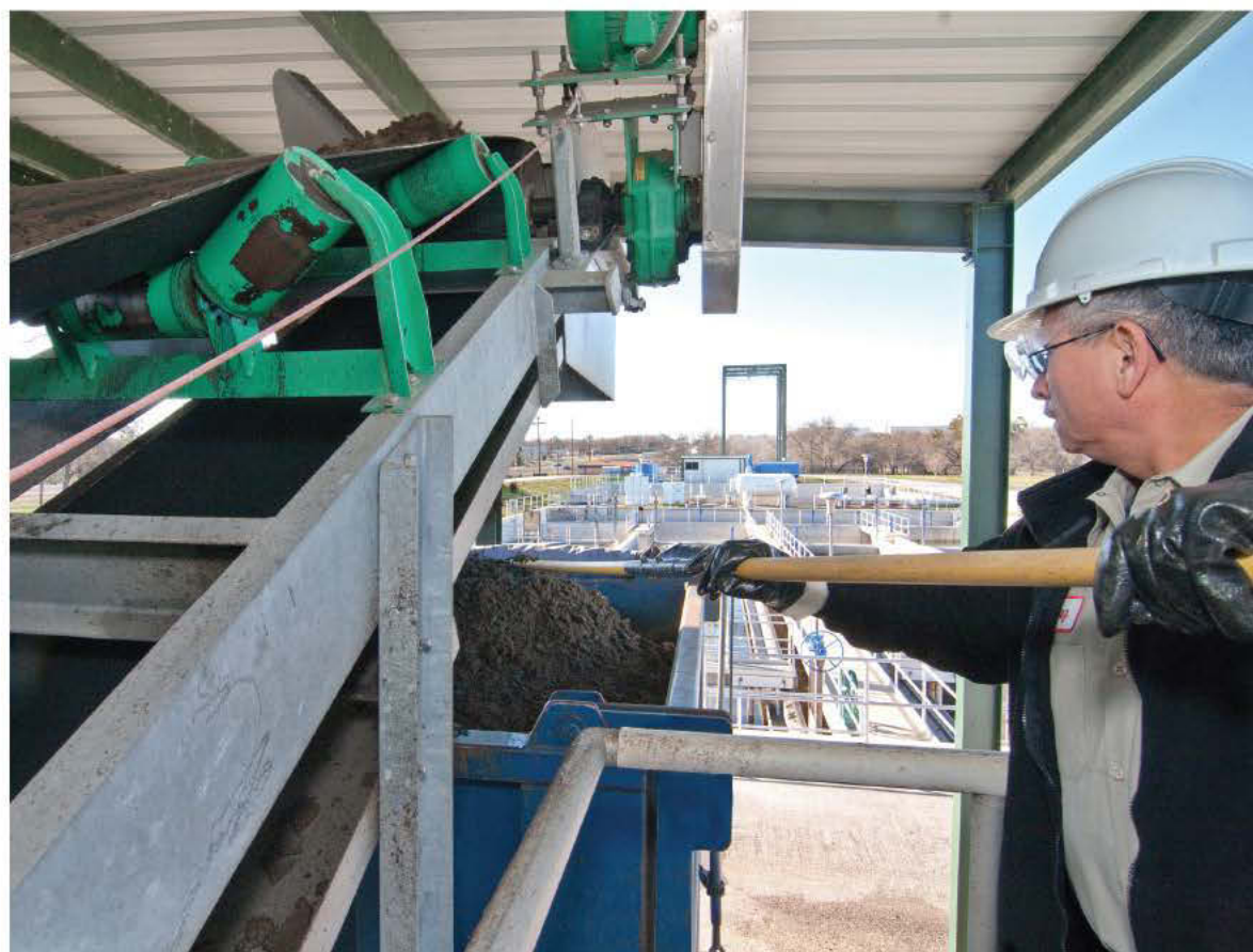
Wastewater operator Cruz Solis evens out the biosolids in a 25-cubic-yard roll-off container (MAC).
