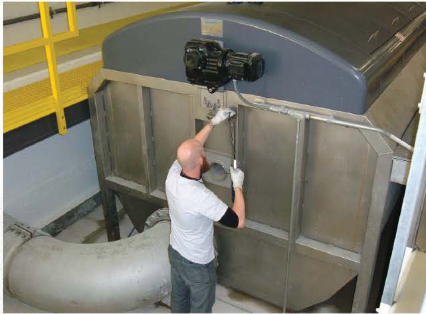
Operator Kevin Kurtz greases one of three drum bearings on a SuperDisc filter.
