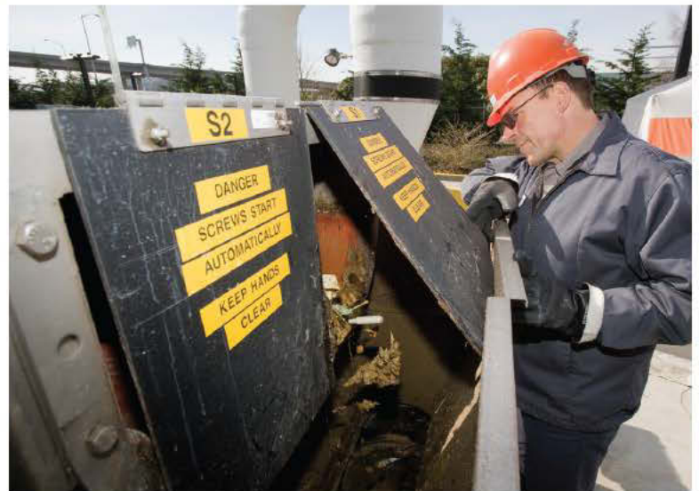
Daily shift operator Bill Shaw at the treatment plant's Mahr bar screens (Headworks).
