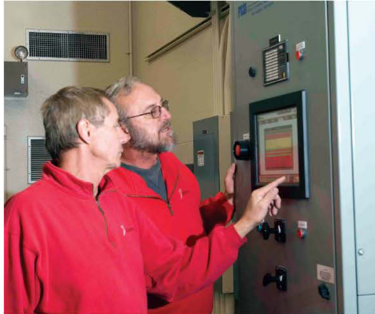
ABOVE: Working foreman/lab technical manager Jim Gauer, left, and maintenance mechanic Paul Marcus monitor the standby generator control panel (Power Systems Solutions). RIGHT: Operator Allen Schueler checks the ferric chloride chemical feed system (Pulsafeeder).
