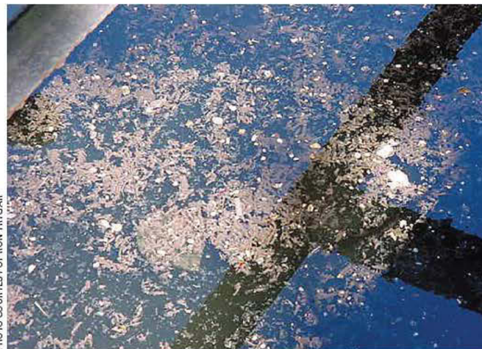
FIGURE 1: Sludge clumps in the aeration tanks looked gray, like shaggy mop heads rising and sinking.
