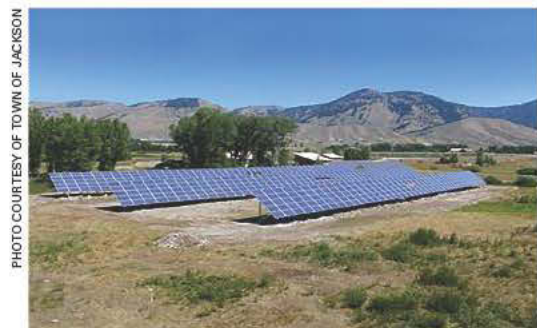
A 165 kW photovoltaic system from Sharp Electronics went live in September 2010 and had generated 16.0 MWh as of March 21, 2012.
