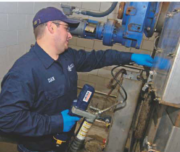
Operator Dan Gehring lubricates bearings on an Aqua Guard mechanical bar screen (Parkson).
