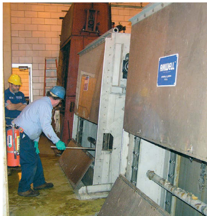
ABOVE: Operator/maintainer II Phillip Minich shows operator/maintainer apprentice Ed Marnon how to access the chain links on the screening system. RIGHT: The chain inspection port is behind a cover that is easily removed for service.
