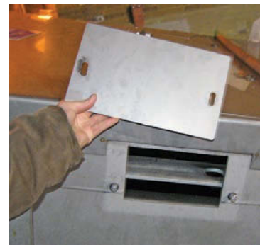
ABOVE: Operator/maintainer II Phillip Minich shows operator/maintainer apprentice Ed Marnon how to access the chain links on the screening system. RIGHT: The chain inspection port is behind a cover that is easily removed for service.
