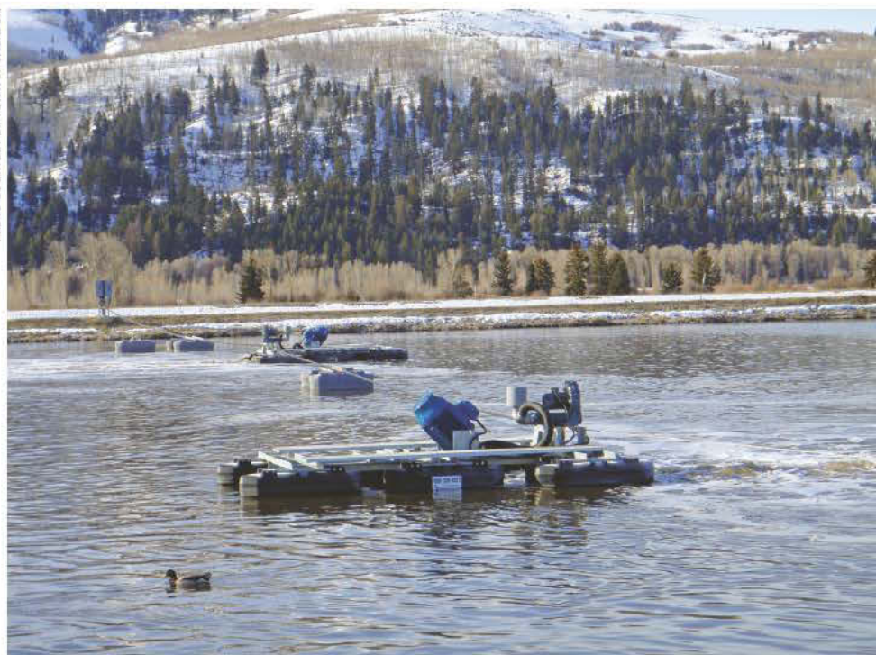
More efficient 50 hp and 25 hp Aire-02 Triton models from Aeration Industries replaced several 75 hp and 40 hp aerator/mixers for surface aeration.
