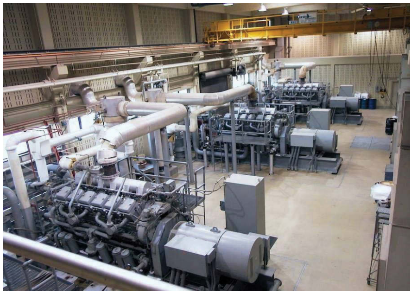
ABOVE: Cogeneration accounts for up to 40 percent of the energy needs of the Wastewater Reclamation Facility in Des Moines. Capacity will increase to more than 50 percent when more engine-generators are added in the near future. LEFT: This main raw water pump is one of six 700 hp pumps at the plant being monitored for energy use.
