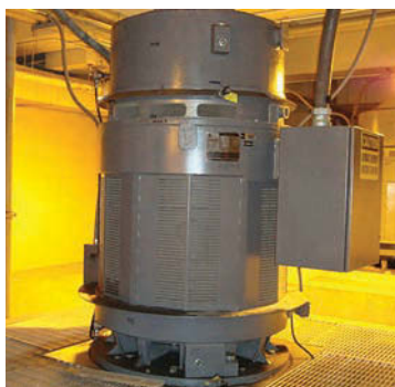
ABOVE: Cogeneration accounts for up to 40 percent of the energy needs of the Wastewater Reclamation Facility in Des Moines. Capacity will increase to more than 50 percent when more engine-generators are added in the near future. LEFT: This main raw water pump is one of six 700 hp pumps at the plant being monitored for energy use.
