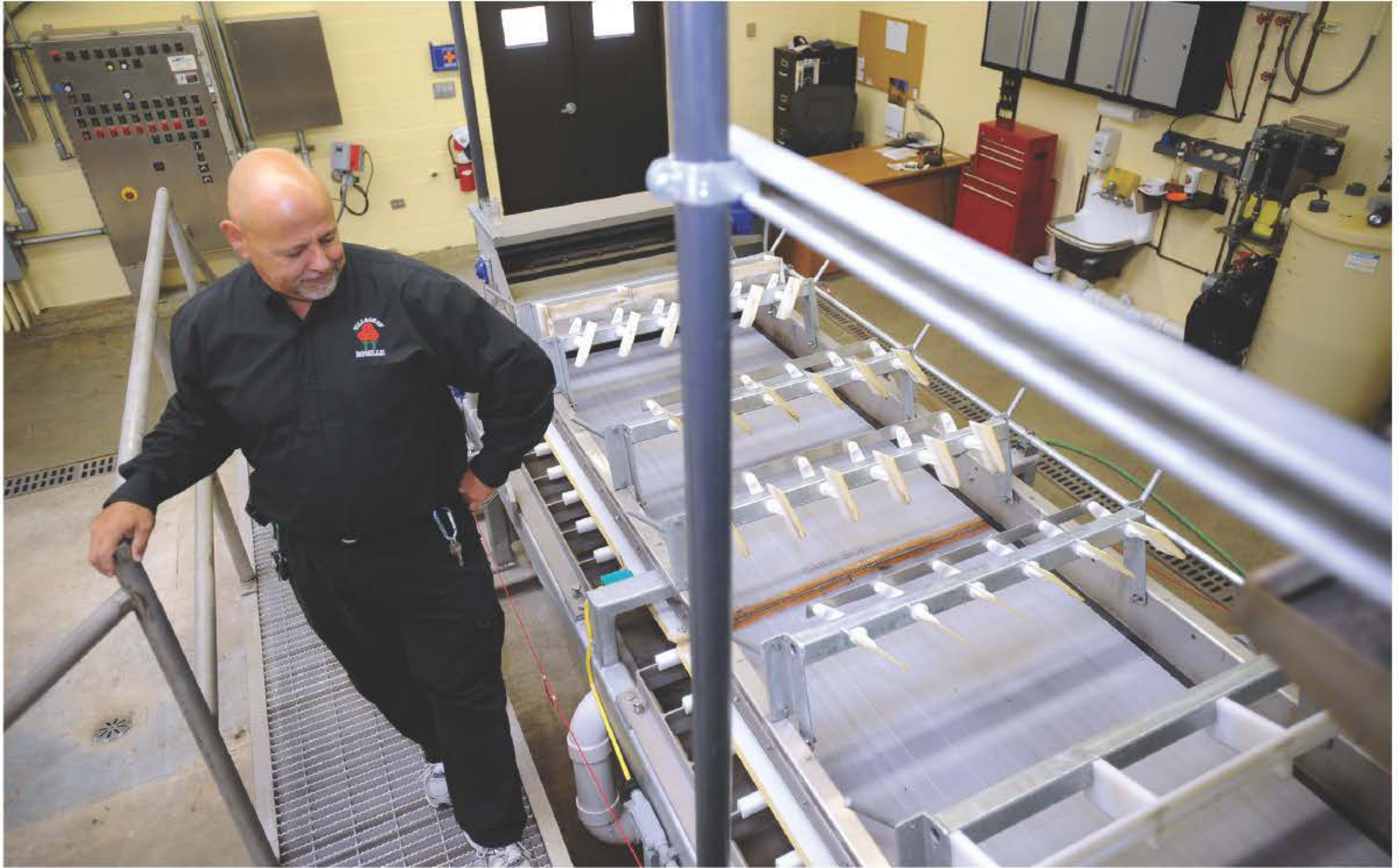
ABOVE: John LaRocca checks on the new sludge press from BDP Industries. BELOW: The Roselle team includes, from left, Botterman plant lead operator Joe Montefalco, collection system operator Jim Campbell, John LaRocca, operator Ron Baird, and Devlin plant lead operator Jeff Peto.
