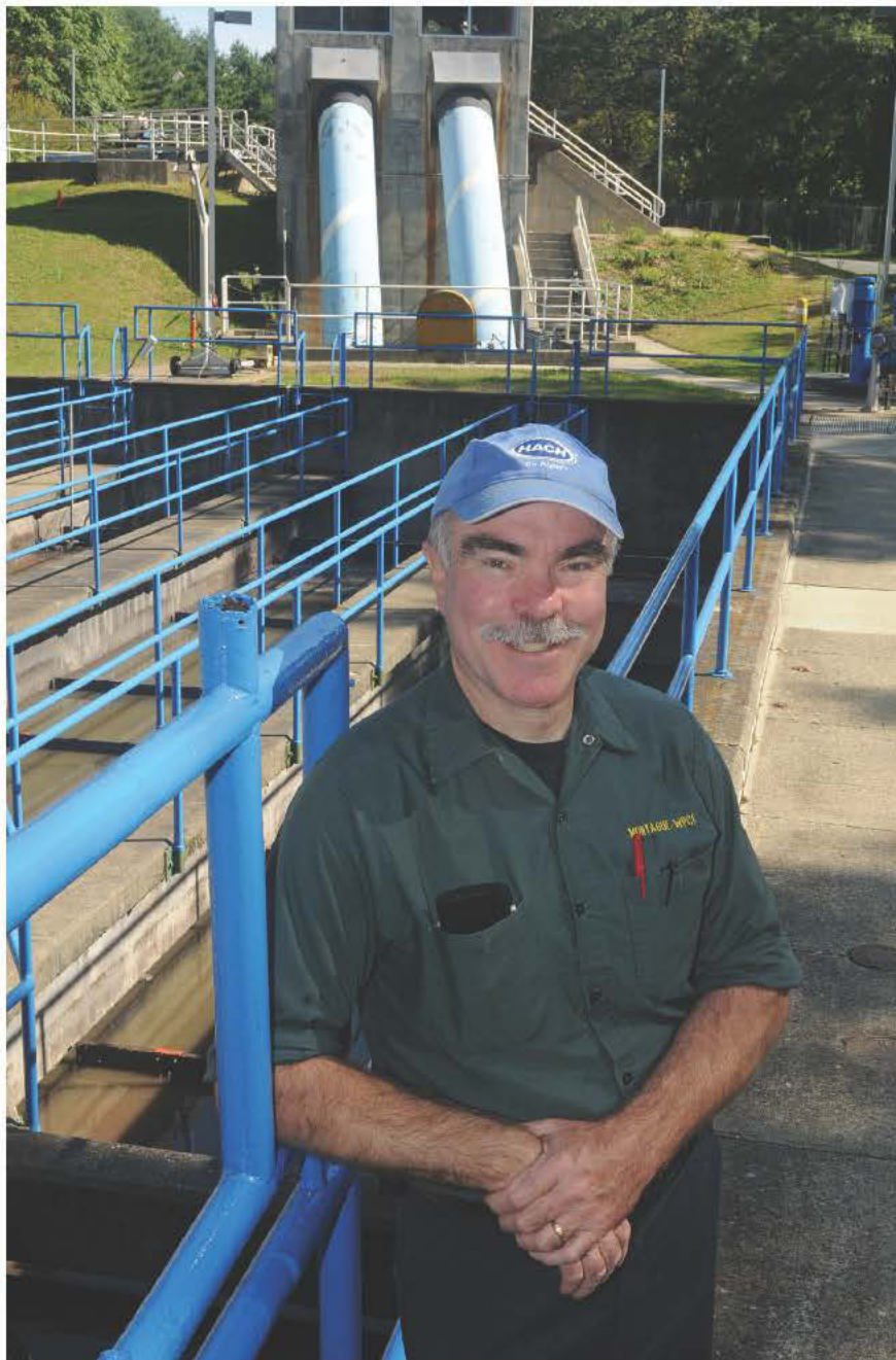
Plant superintendent Robert Trombley and his team added effective CSO treatment and made other improvements at the Montague facility.
