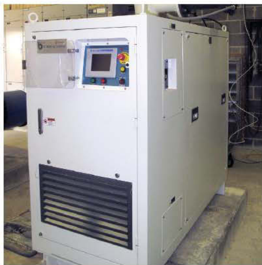
Unit 3 in the blower room at Longview's Grace Creek Wastewater Treatment Plant is a new APG-Neuros NX 150 aerator blower that can be used to supply air to any of the four aeration basins at the facility.
