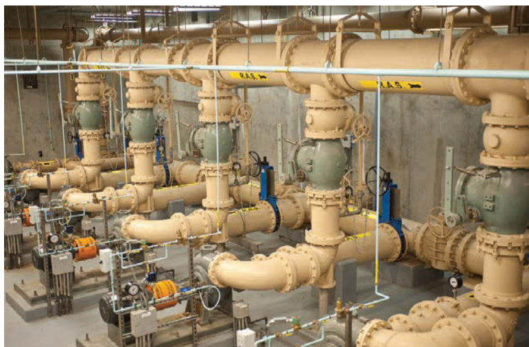
The plant uses pumps from Flygt – a Xylem brand, for return activated sludge (RAS) and waste activated sludge (WAS).
