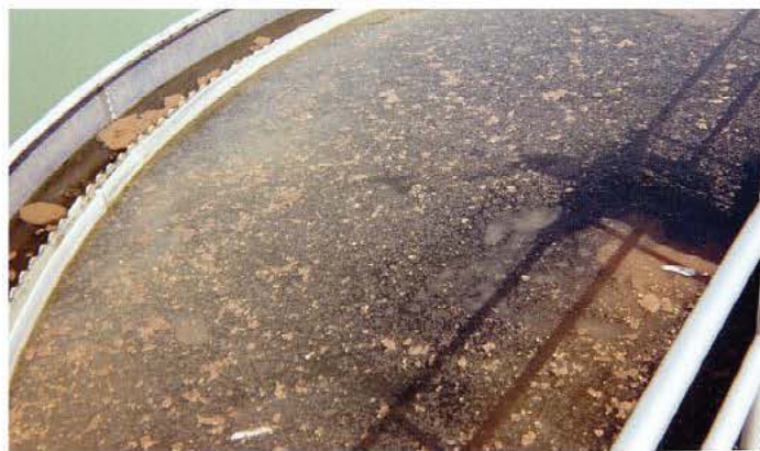
FIGURE 1. Solids rising and extending across the clarifier surface. (Photo by Ron Trygar)
