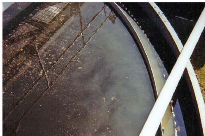
FIGURE 2. White, cloudy effluent leaves the secondary clarifier. (Photo by Ron Trygar)
