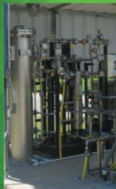
Biogas Conditioning System and Capstone Turbine at Grace Creek Wastewater Treatment Plant in Longview, Texas
