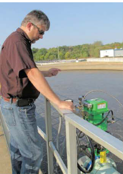
Scott Baggett, plant manager at Longview's Grace Creek Wastewater Treatment Plant, looks at one of the new pneumatic actuated K-Tork butterfly valves that help operators maintain the proper airflow in the plant's four aeration basins. (Photos by Pete Litterski)
