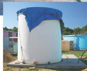
ABOVE: The EcoFilter EF 124 biotrickling reactor for the sludge storage tank and rotary drum thickener at the Rancocas Road facility has a 4,800 cfm blower.
