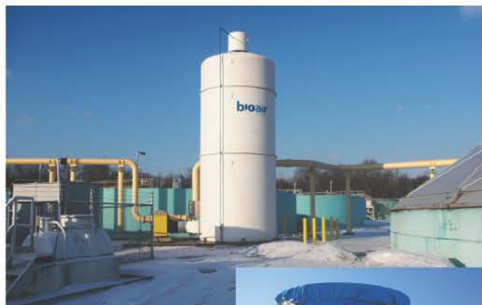
ABOVE: The EcoFilter EF 124 biotrickling reactor for the sludge storage tank and rotary drum thickener at the Rancocas Road facility has a 4,800 cfm blower.
