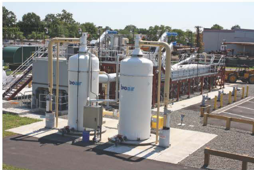
The Maple Avenue facility has two EcoFilter EF 62 biotrickling reactors with 1,030 cfm blowers controlling odors from the headworks.
