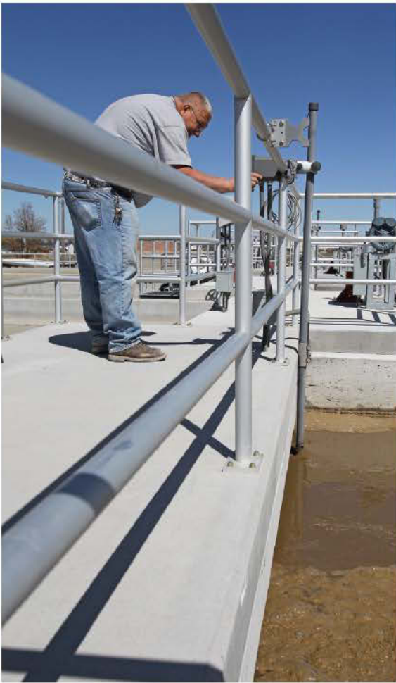
LEFT AND ABOVE: Ralph Martini checks the oxygen levels in the activated sludge process.
