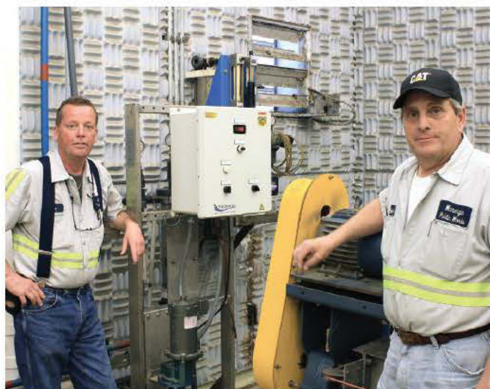
ABOVE: Operator Tim Mack, left, and Jay Berman, superintendent of the City of Marengo Wastewater Treatment Facility, use the dynaBLEND liquid-polymer activation and blending system from Fluid Dynamics, a division of Neptune Chemical Pump Co. RIGHT: The processed biosolids material is eventually used as fertilizer.
