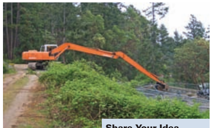
By cleaning the media in place rather than replacing the gravel in the filters, the Eastsound Sewer and Water District saved money and labor.
