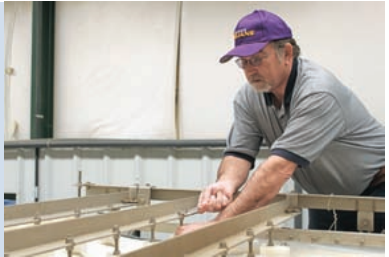
Larry Tignor, Class 4 operator, adjusts the dividers on a belt filter press from OR-TEC. (Photography by Dianne Saison)
