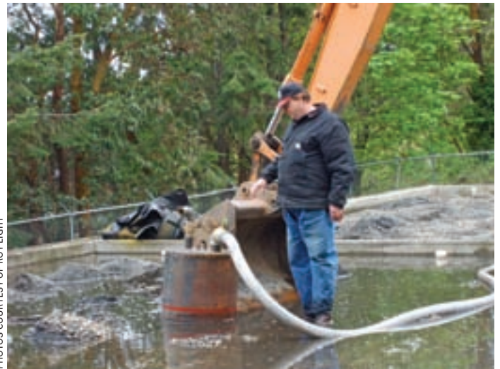
Eastsound Sewer and Water staff devised a plan to push a 6-foot-tall by 2-foot-diameter cylinder into the gravel while applying vacuum to fluff the gravel and draw the sludge into the truck for disposal.
