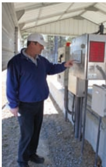
Frankie Sanders, assistant supervisor and Class 1 operator, checks the UV disinfection system (Trojan Technologies).
