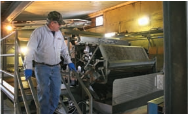
ABOVE: Operator Randy Oesch operates the Ashbrook Klampress belt press. RIGHT: Samples are taken at the aeration basin to measure the ORP/pH balance.
