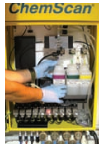
Maintenance is performed on the facility's ChemScan denitrification analyzer.
