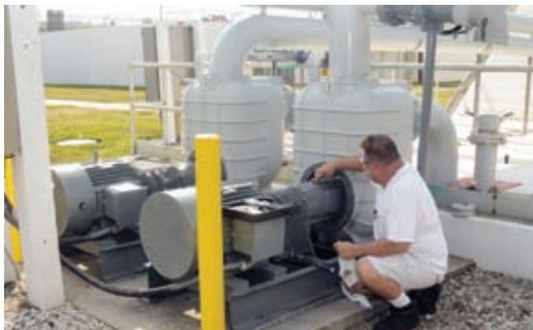
Kelly Frazier, day shift lead operator, changes the oil on one of the plant's tandem aboveground pumps from ITT Water & Wastewater.
