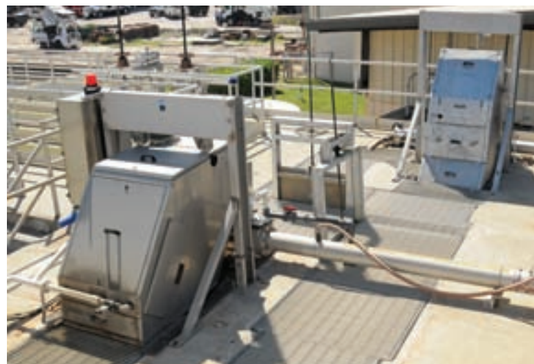
Influent screens from Huber Technology are part of the headworks at Tarpon Springs.
