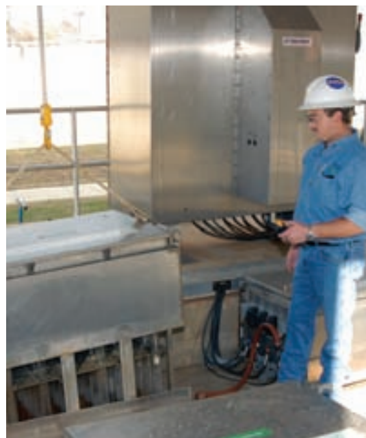
Operator Chris West pulls a UV module from the Ozonia disinfection system for maintenance.
