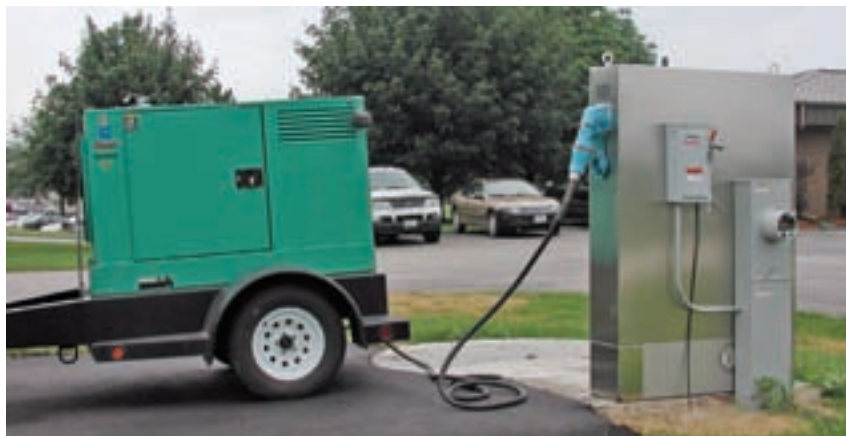
The Decontactor provides a safe connection between the generator and lift station.
