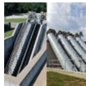
Tube-Mounted Screw Pump and Open-Flight Screw Pump from Schreiber
