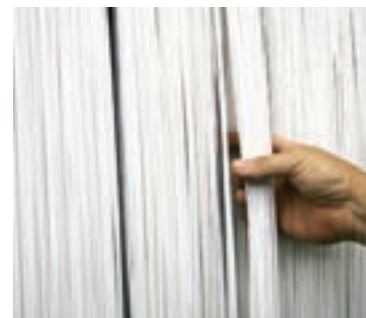
RIGHT: The ZENON membrane basins are the heart of the facility. The membranes are hollow strands of porous plastic fibers.
