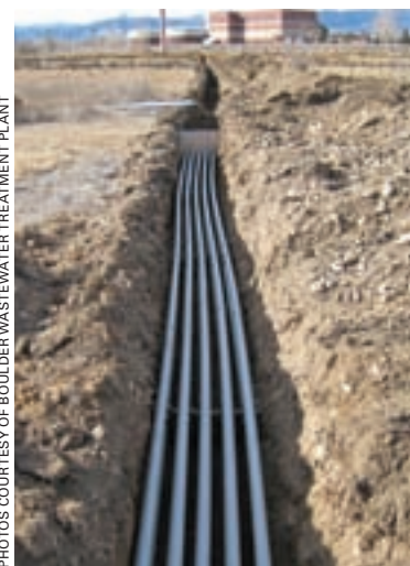
Underground lines lead from the 1 MW solar photovoltaic systems to the Boulder Wastewater Treatment Plant.
