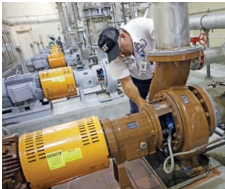
ABOVE: Maintenance technician Jim Davis performs routine service on Gardner Denver centrifugal blowers.
