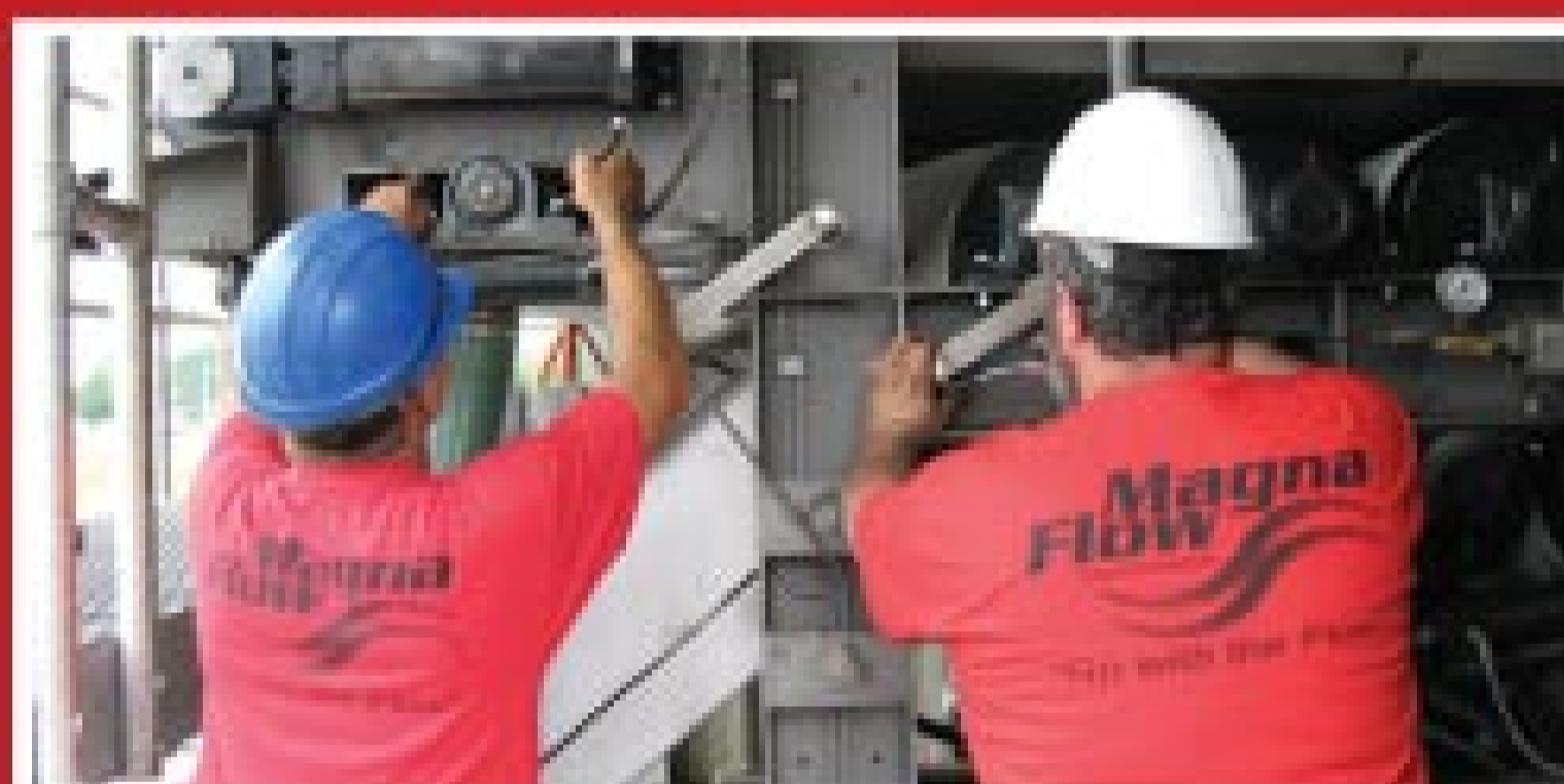
Belt Press Repair & Maintenance
