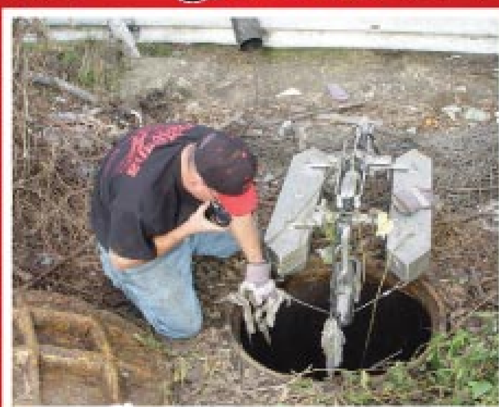
Large Diameter Pipe Inspection
