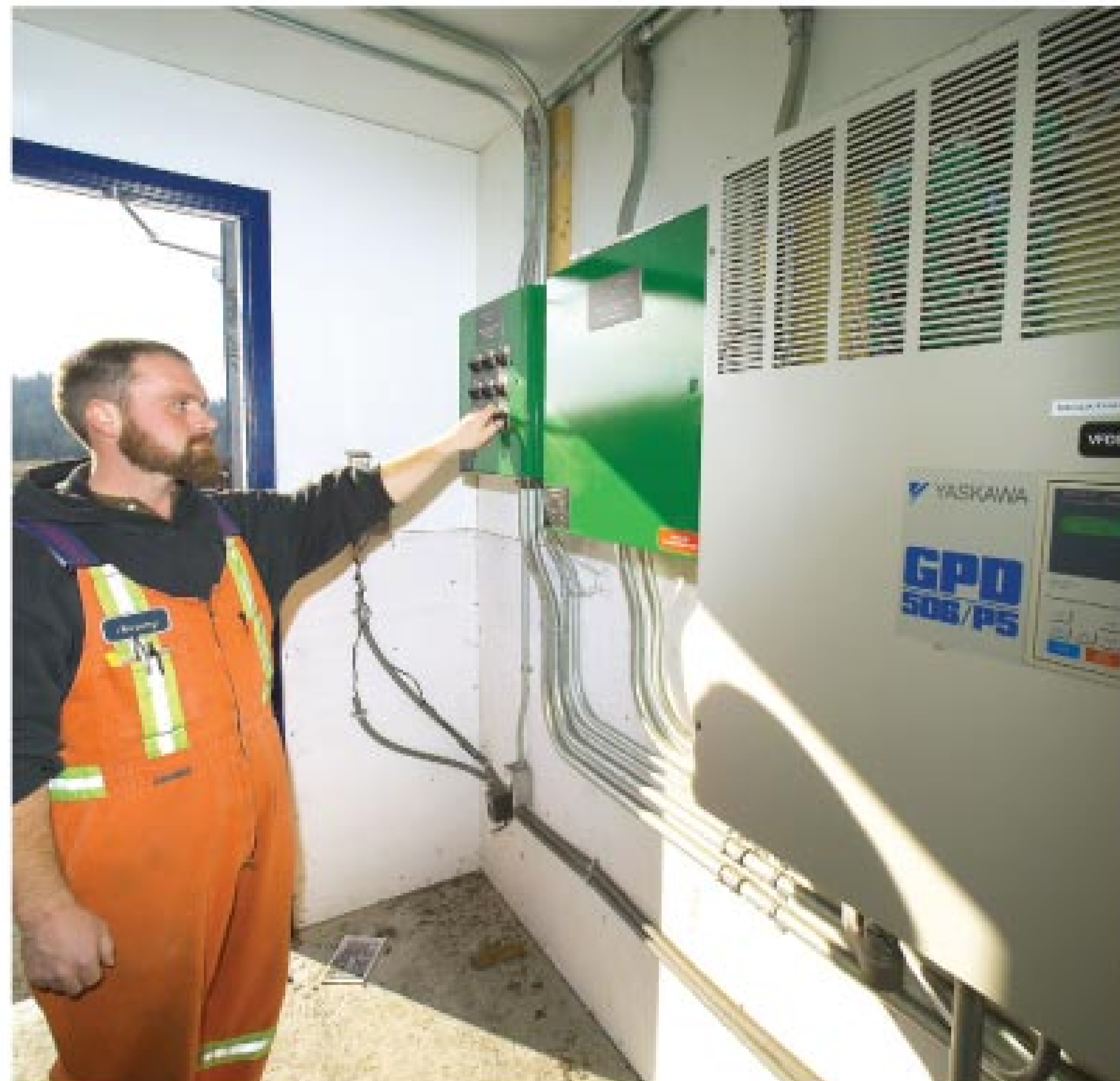
Jeremy Kozub adjusts the volume of airflow to the compost piles. The air is delivered via blowers with a drive from Yaskawa America.
