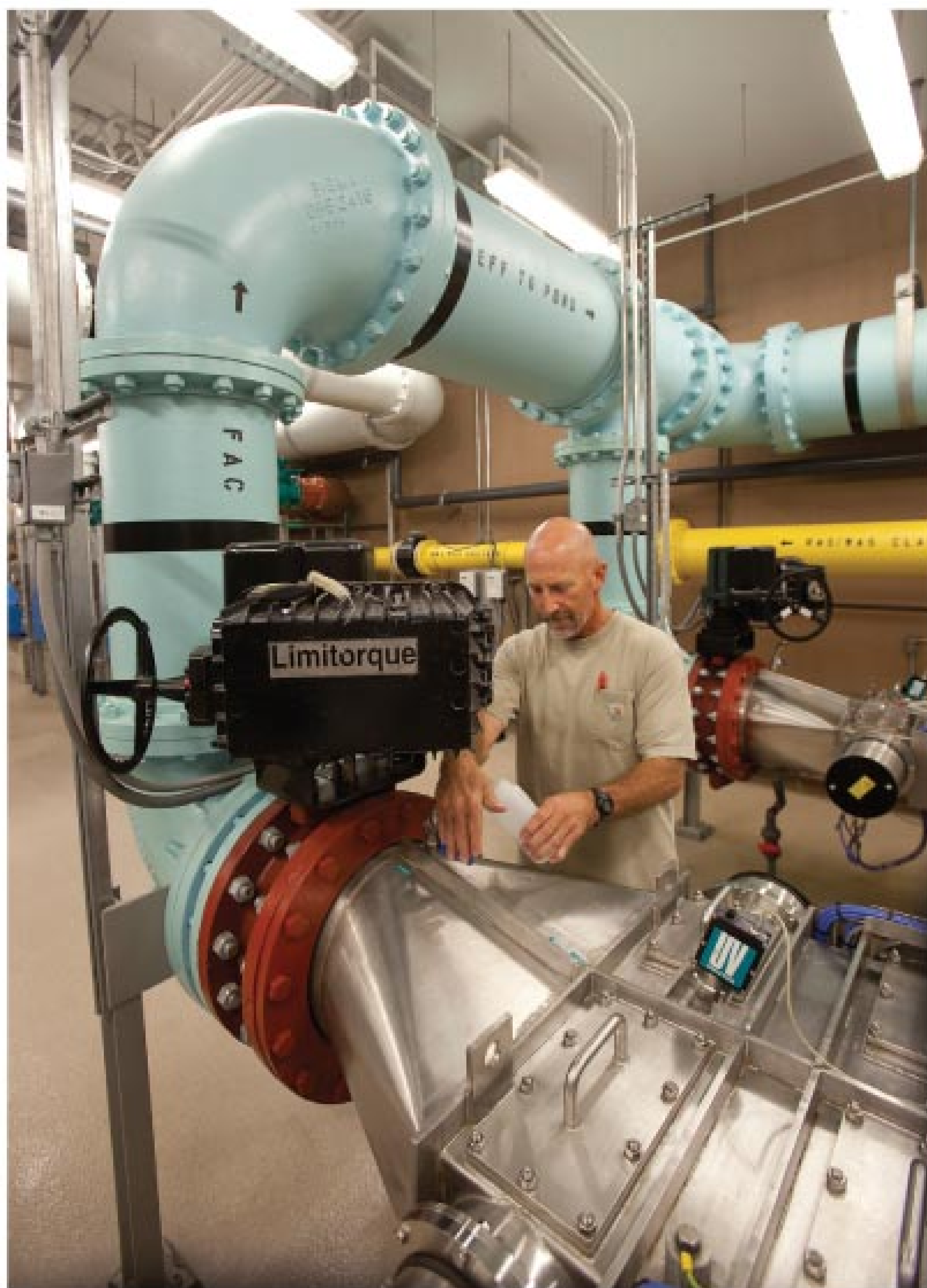
ABOVE: Class 4 operator Pat Fountain takes one of the daily water samples used to check for E. coli and other bacteria, as well as ammonia. LEFT: A Royce handheld TSS meter is used to test for mixed liquor suspended solids in the aeration basin.
