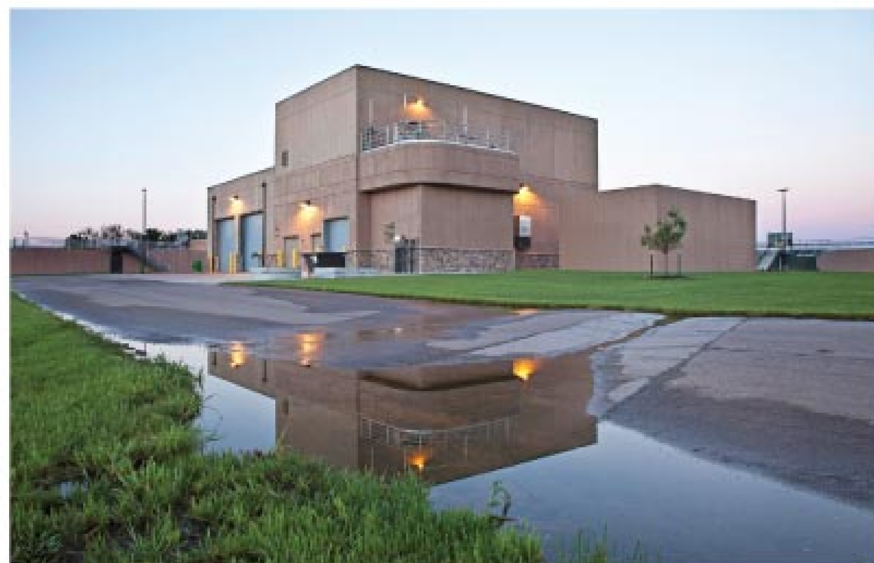
The El Dorado Wetlands and Water Reclamation Facility.
