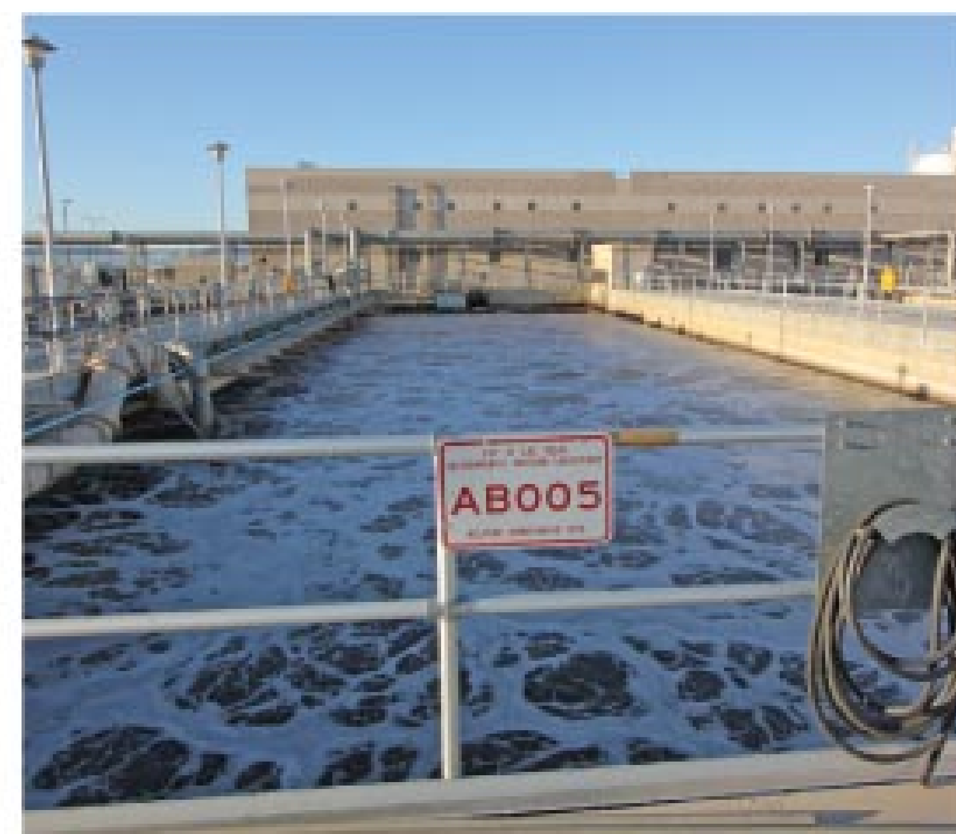
The nitrification aeration basin at the Las Vegas treatment facility.
