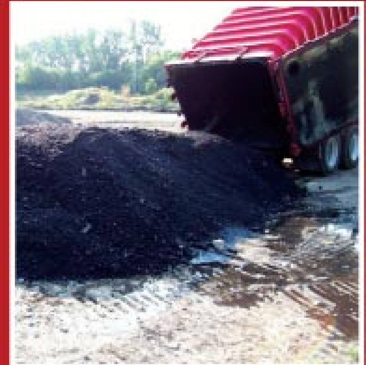
Paint Filter Dry Material Removed From Sewer Line
