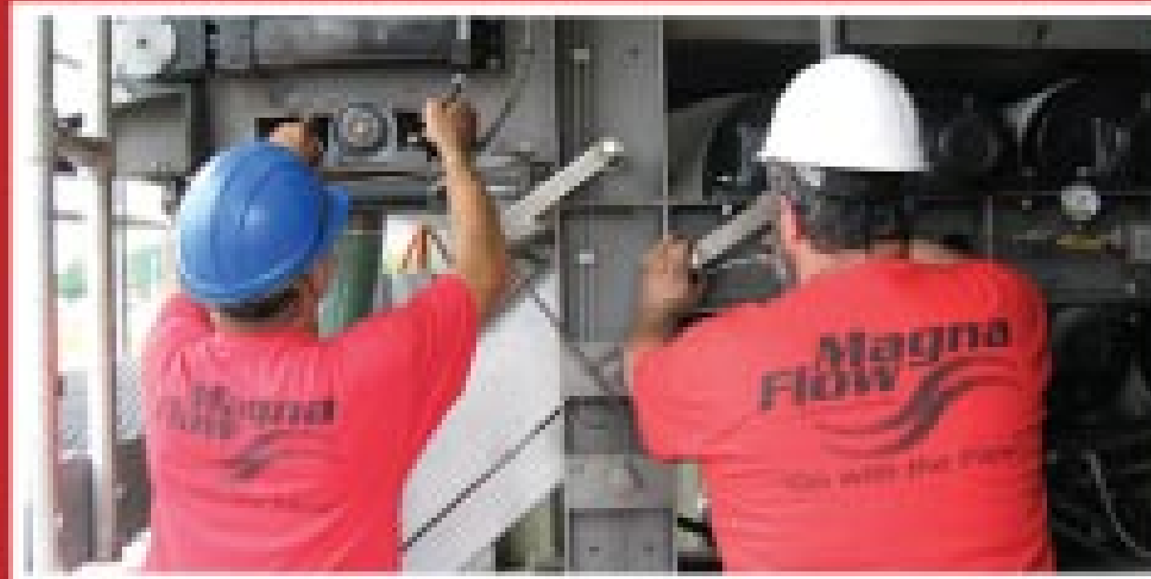
Belt Press Repair & Maintenance
