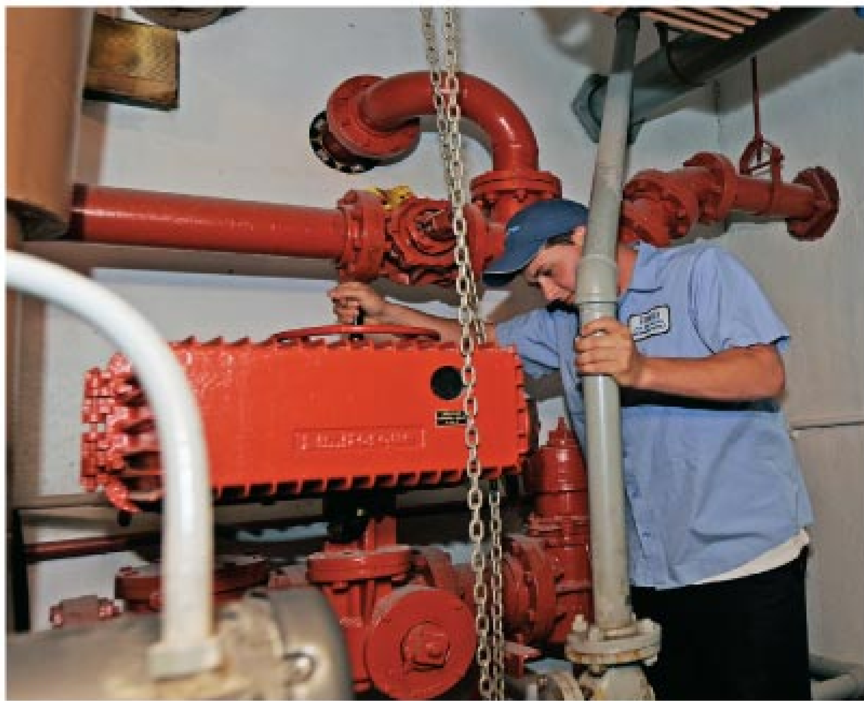
Phil Miller maintains the sludge and oxygen levels in the aeration tanks.
