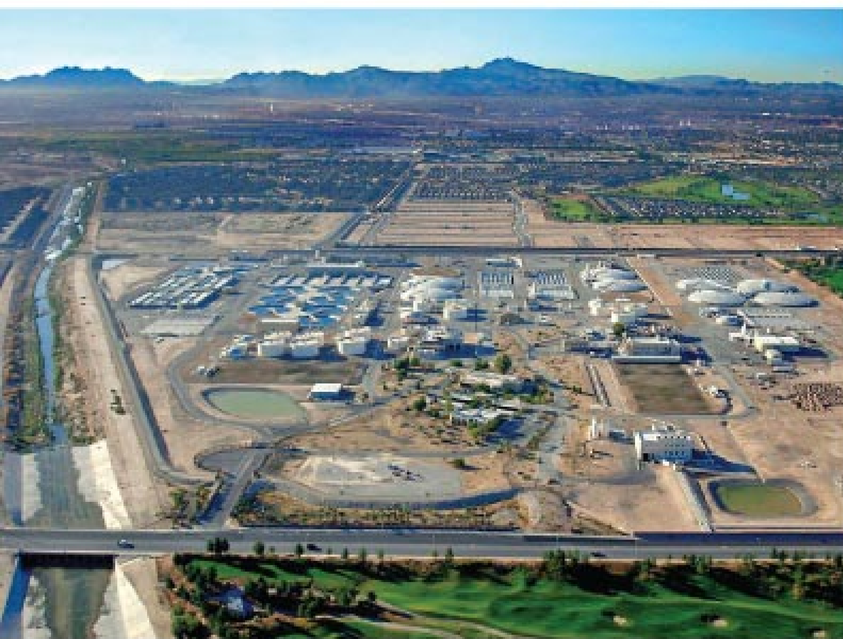
The Las Vegas Water Pollution Control Facility treats 65 mgd of wastewater for people in Southern Nevada. Treated water is discharged to the Las Vegas Wash (left) and flows to Lake Mead. Some treated water irrigates two neighboring golf courses.
