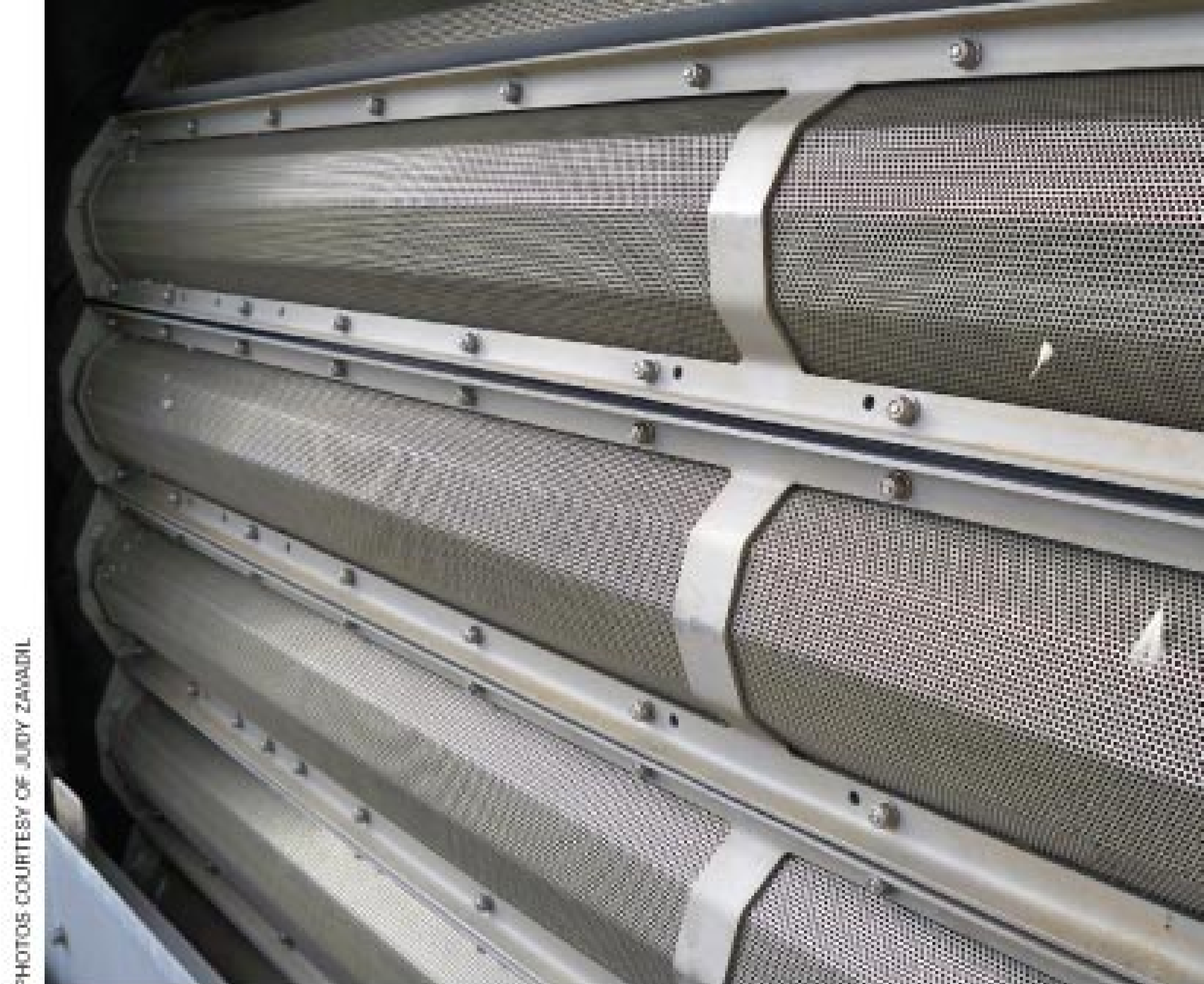
Rows of rotating stainless steel sieves with 2 mm holes on the Eliminator band screen from Headworks capture plastic bits, grease balls, and the occasional feather.
