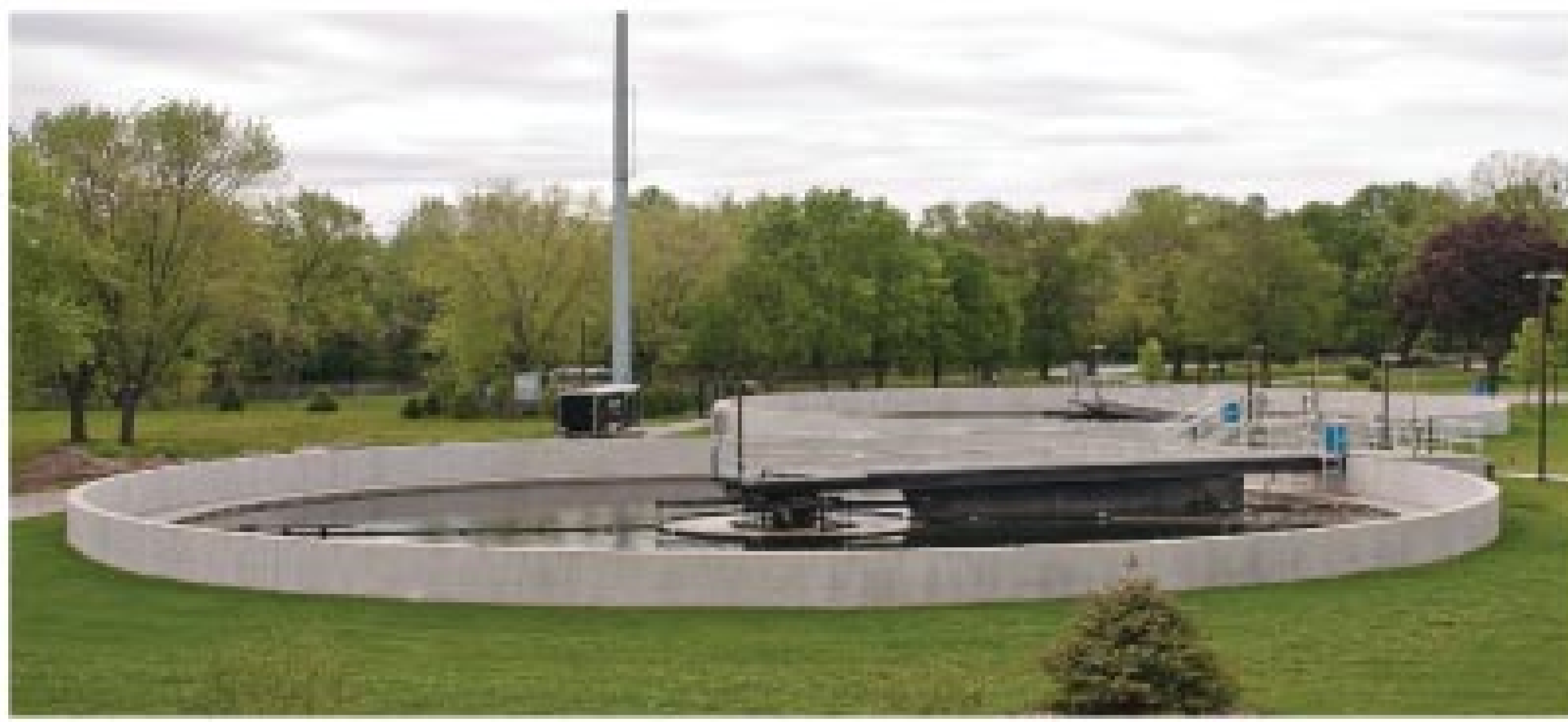
ABOVE: One of the two final Envirex Tow-Bro circular clarifiers. BELOW: The plant's SCADA system, which includes PLCs from Allen-Bradley (a division of Rockwell Automation) and Intellution software. The system provides monitoring and control at five locations within the plant as well as on staff laptops.
