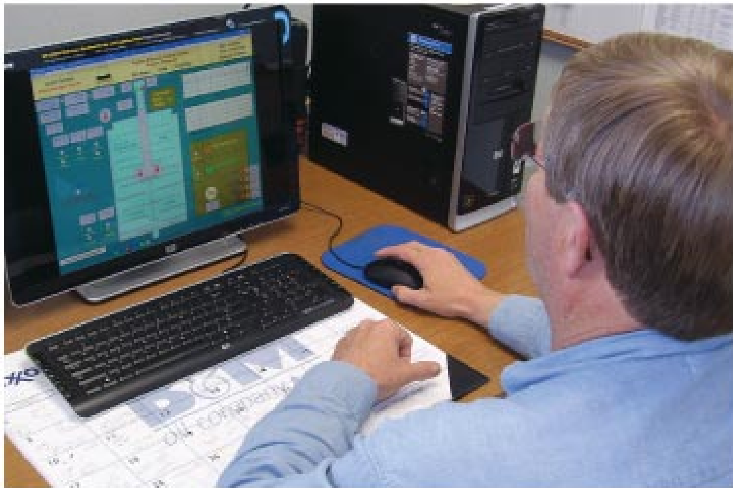
Operations manager Robert Moore monitors instrumentation data on the plant's control system.
