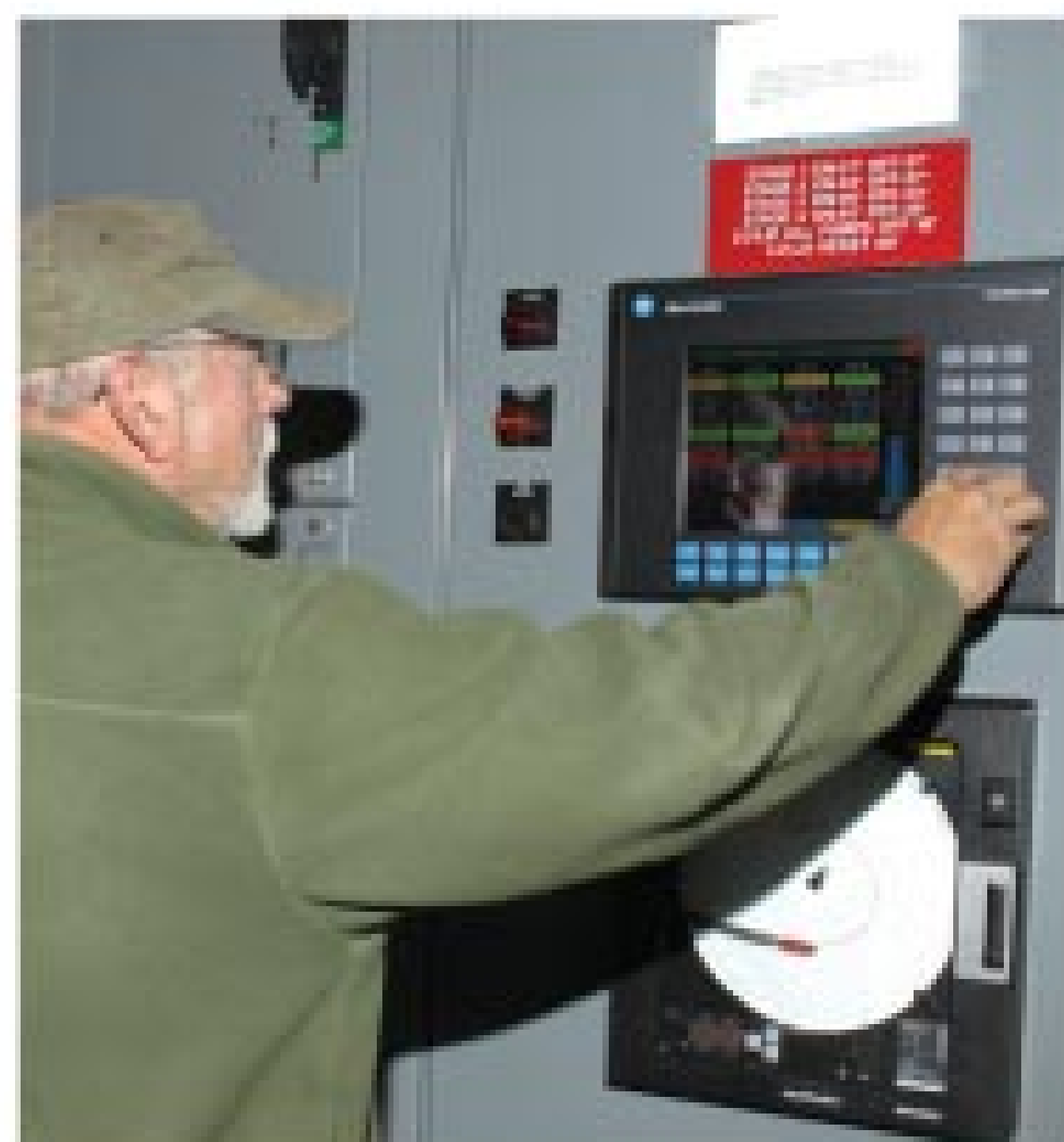
Rich Crane, electronics technician, observes the operation of equipment controlled by Allen Bradley Panel View PLC.
