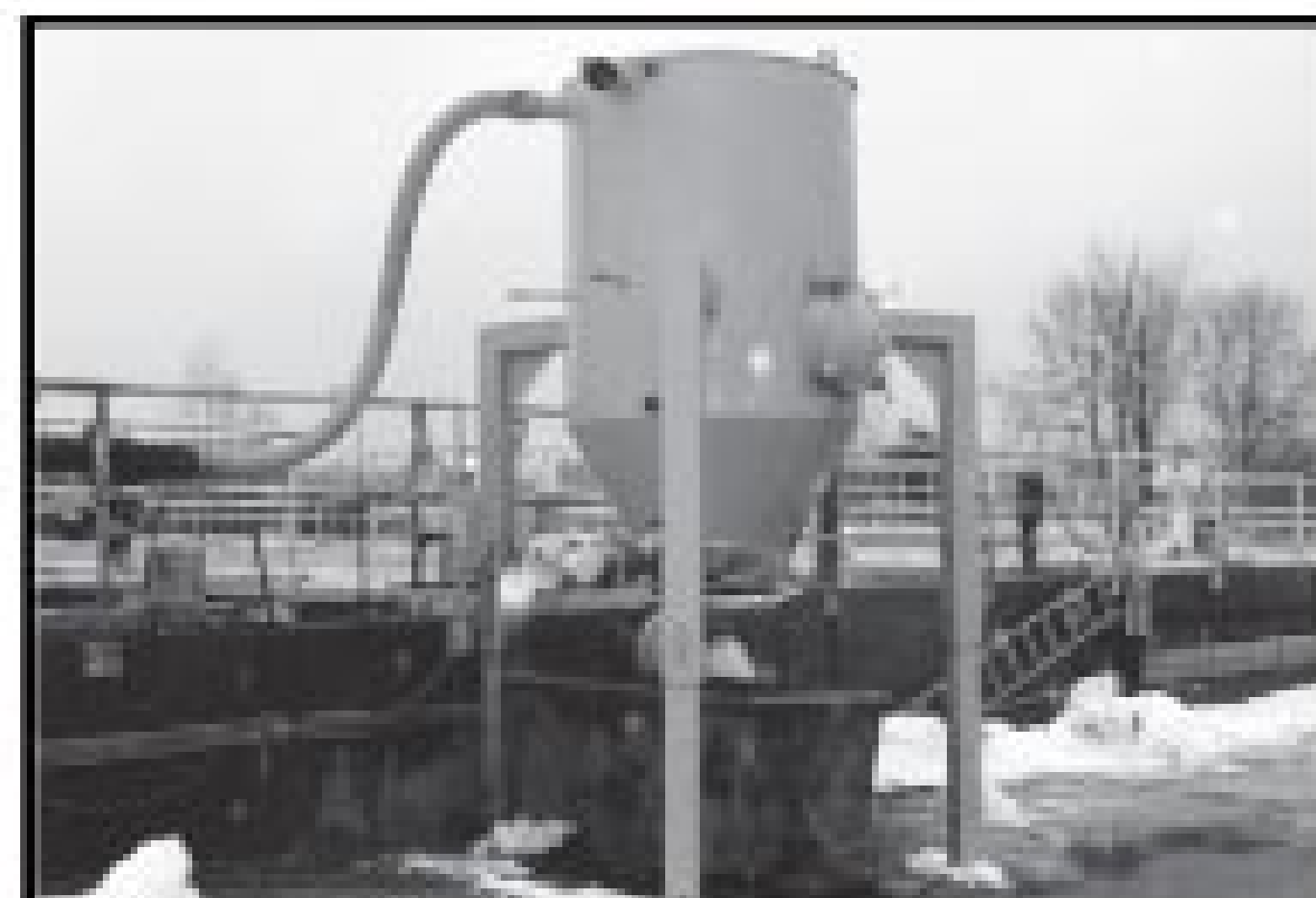
Grit Grabber 750 : Catches the grit to keep it from entering into the Waste Water Treatment Plant or storage tanks. $21,000 603-428-3351 OB
