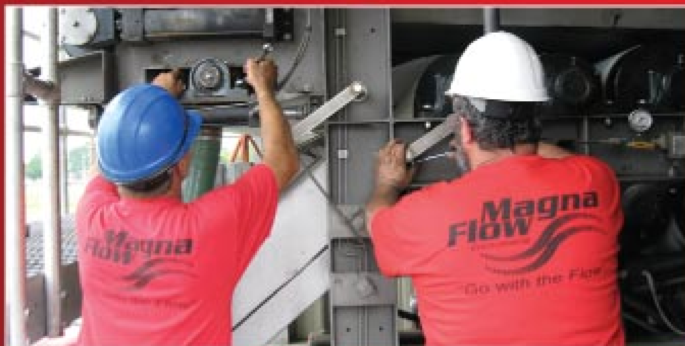
Belt Press Repair and Maintenance
