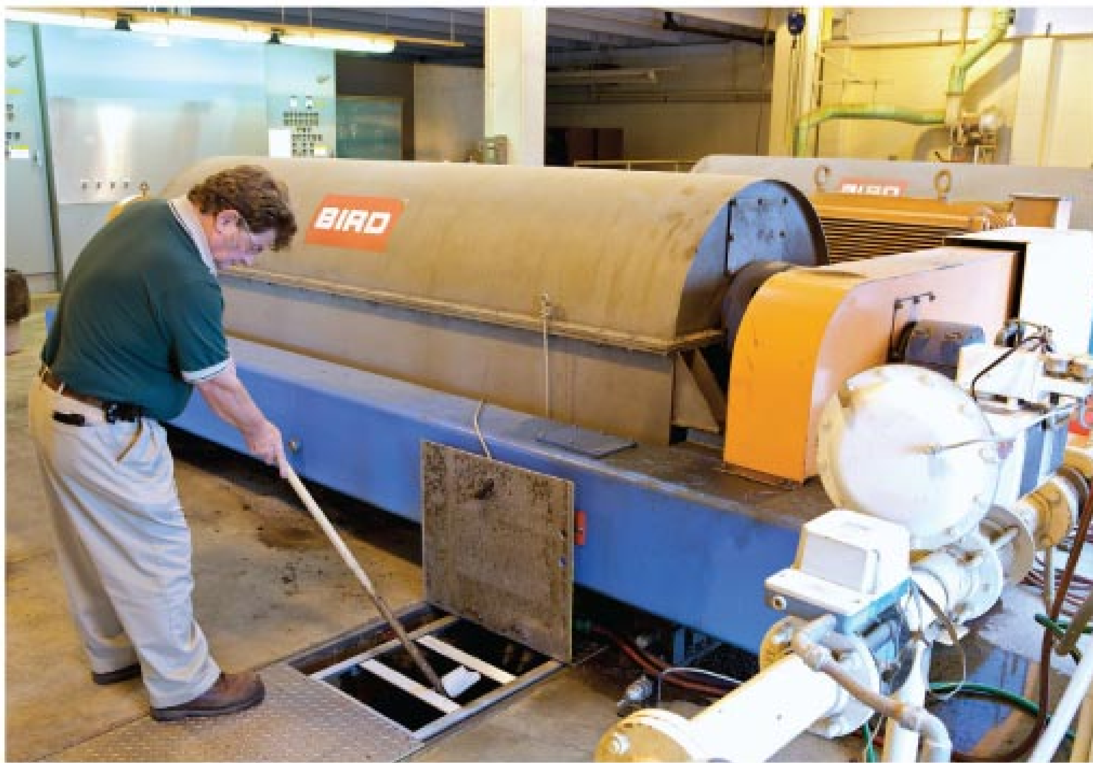
LEFT PHOTO: Utility plant operator Don Uitulugt checks cake from a Bird Humboldt (Andritz Separation Inc.) centrifuge at the Wyoming facility. ABOVE: Ron Kryger, utility plant operator, visually checks the cake level in a hopper with a Siemens Energy & Automation meter at the Grand Rapids facility.
