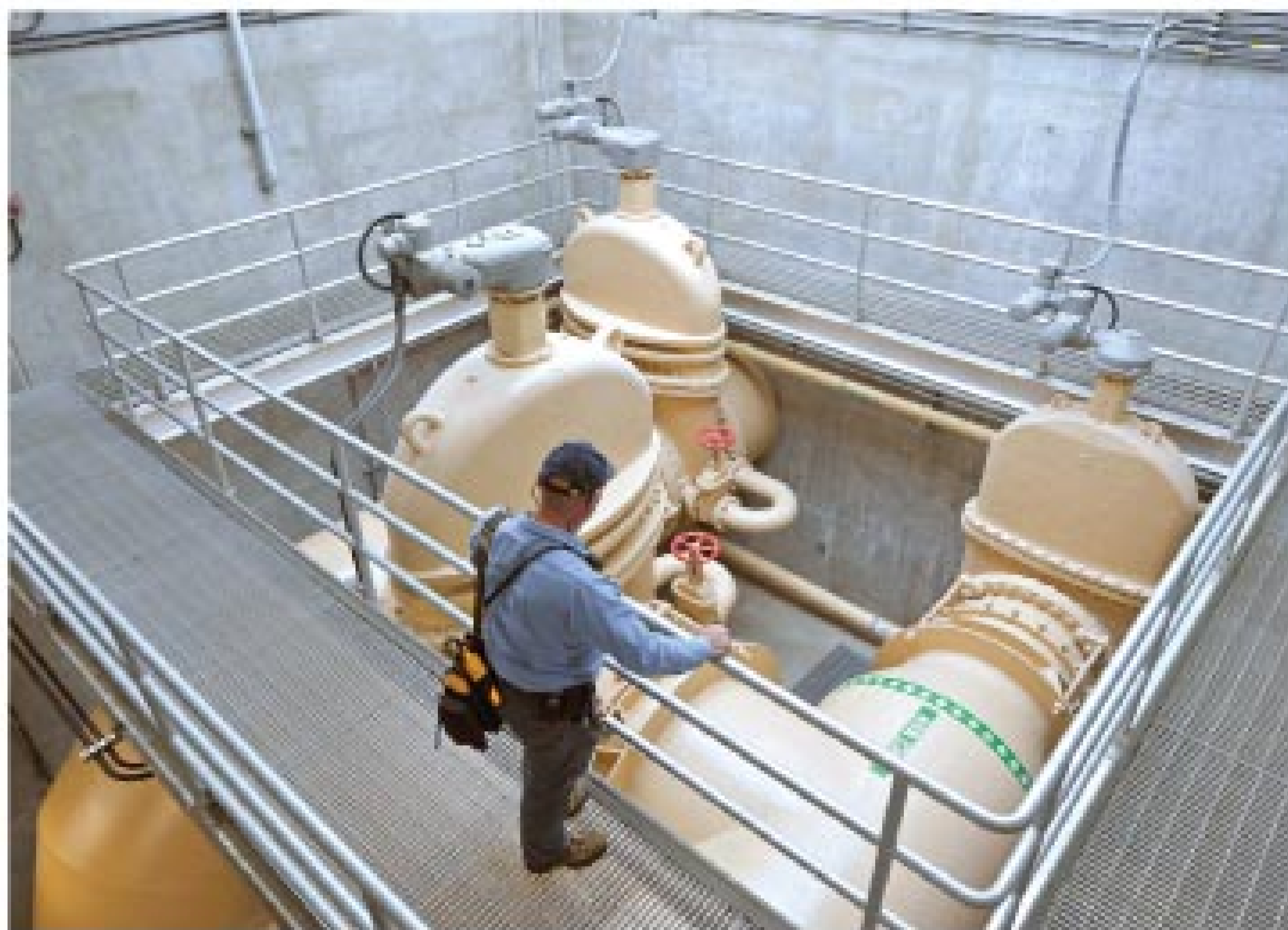
Jeff Keikkala, a plant instrument technician with Clean Water Services, inspects the Neo Seguro valves that direct flow from the influent pump station to the force mains that lead to the headworks.
