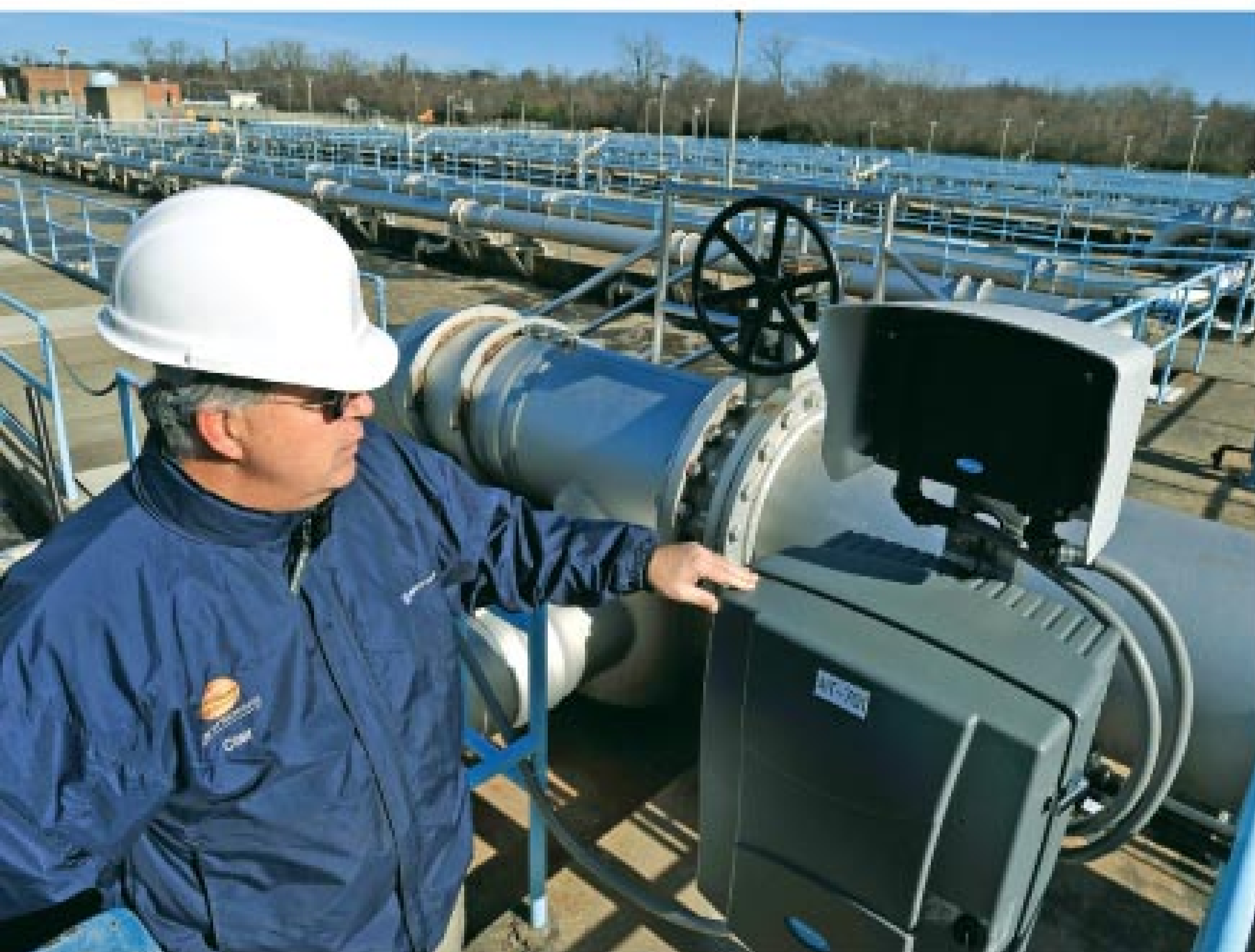
ABOVE: Bernard Evans, operator/maintenance technician, checks the raw sewage pump control station at the front end of the treatment plant. The plant's management information system (Invensys Operations Management - Foxboro) appears onscreen. LEFT: Clair Watson looks at an in-progress installation of a Hach nutrient analyzer in the aeration tank section of the plant.
