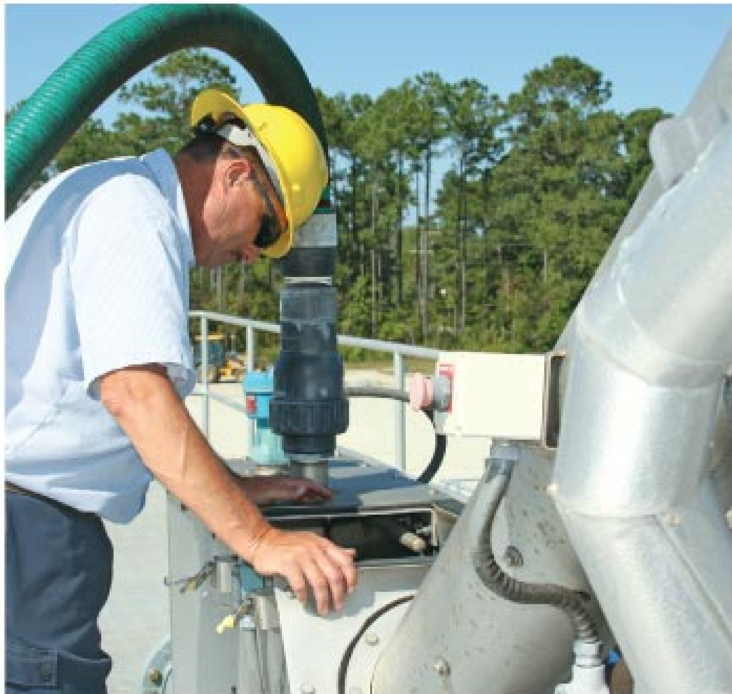
Dale Richmond checks the influent screen at Summerhouse for proper function.
