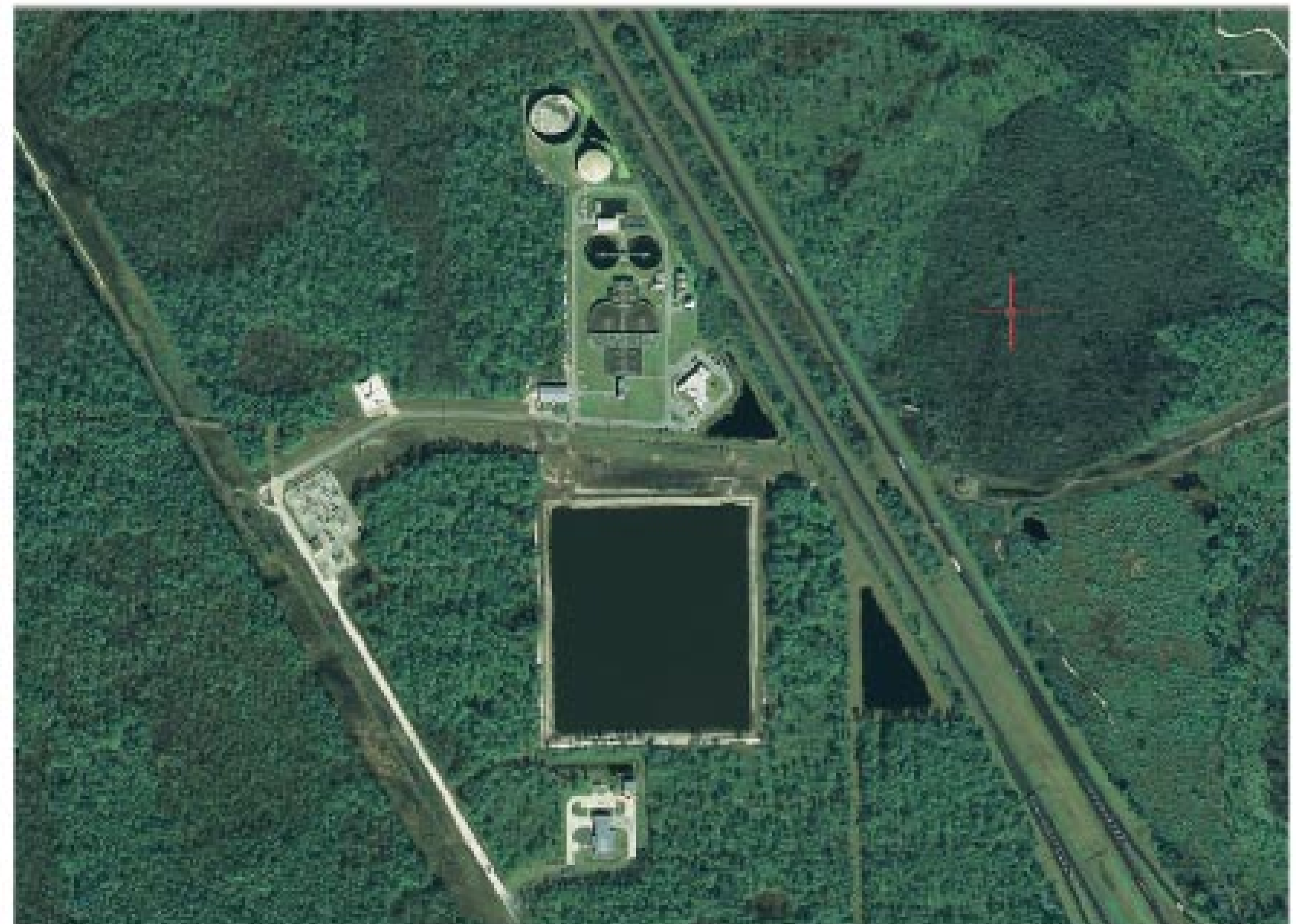
The 13-acre reuse pond was instrumental in enabling more reuse rather than discharging water to the ocean outfall.
