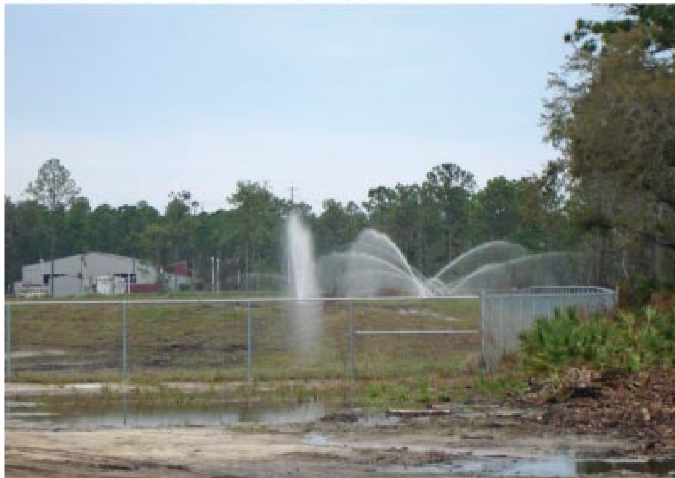
This view looks south from the New Smyrna Beach plant toward the 13-acre reuse pond and irrigation area. Investing in the pond and irrigation helped reduce loss of water and energy to pump to the facility's river outfall five miles away.
