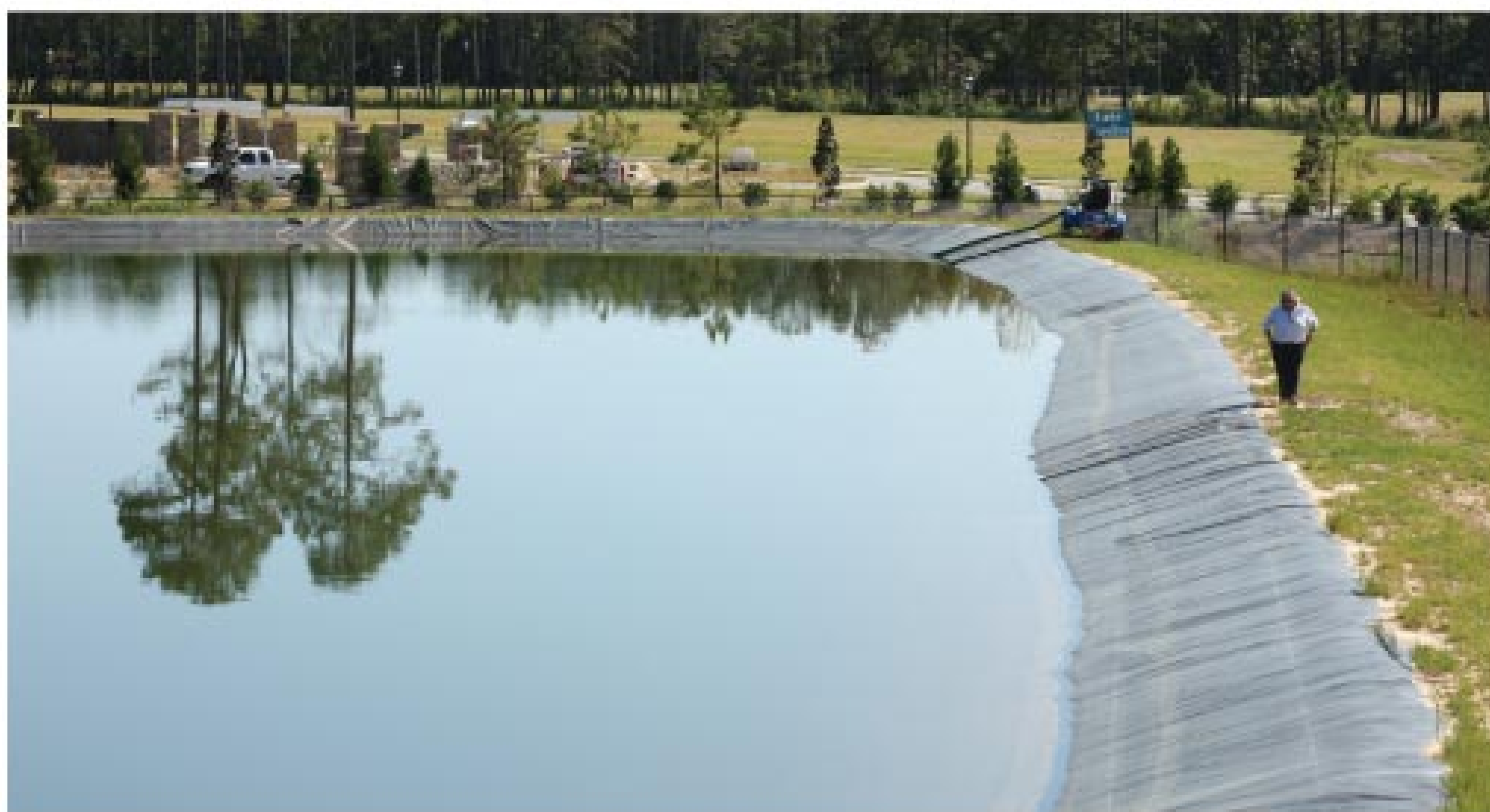
Facility superintendent Karen Wallace surveys the upset lagoon at the Summerhouse Water Reclamation Facility, which provides for the agency while reducing demand on potable water supplies. (Photography by Erica Conner)
