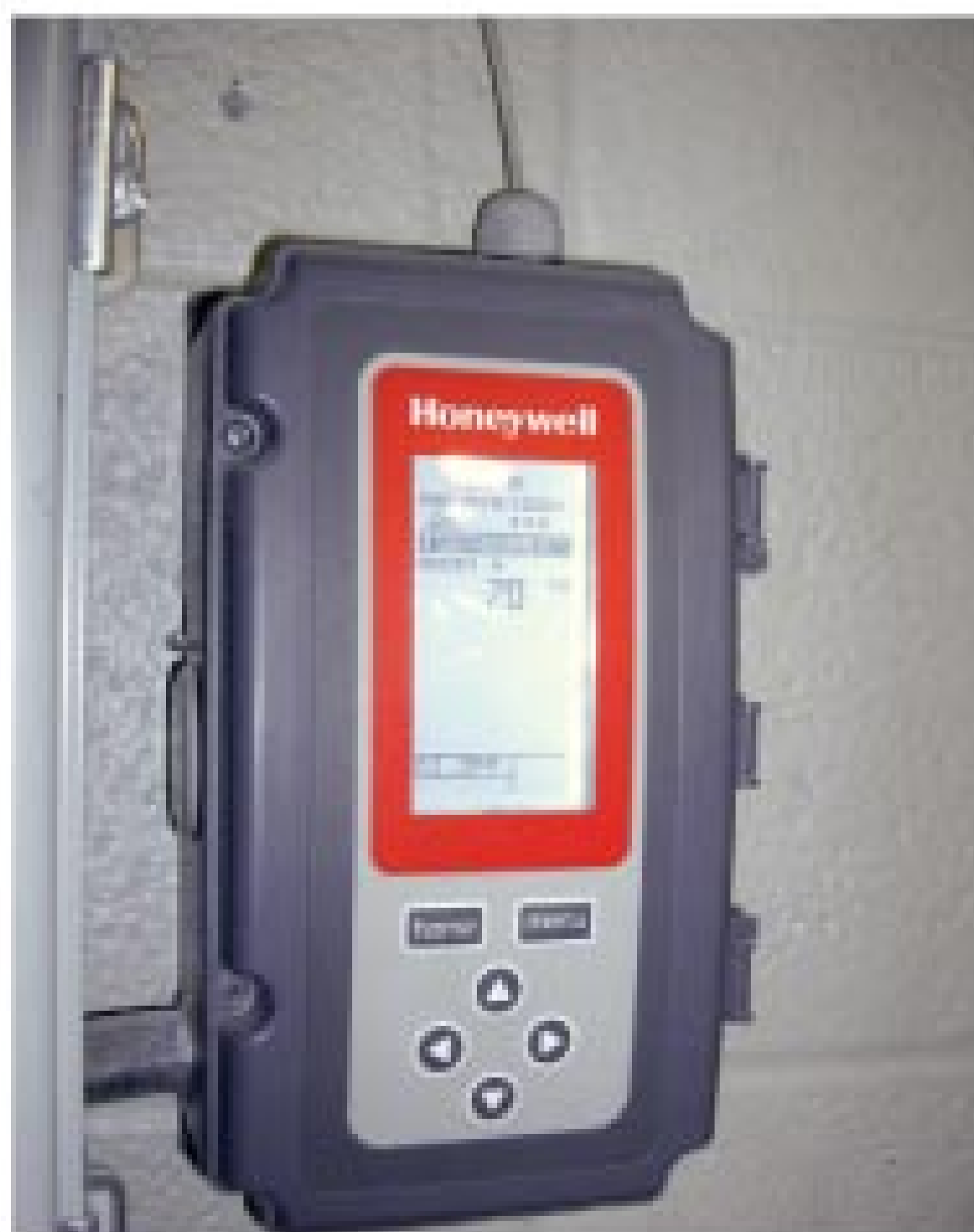
A programmable thermostat is one way to keep control of heating costs.
