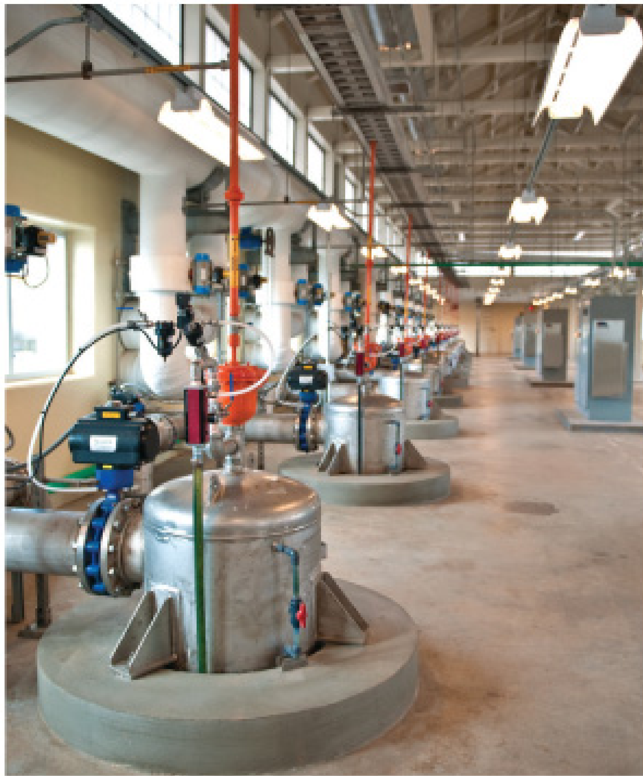
ABOVE: a 12-train ZeeWeed 500 membrane system from GE-Zenon. CENTER: James Marrone performs a calibration on a sodium hydroxide (caustic soda) pump. Right, Marrone with the plant's odor scrubber tower.
