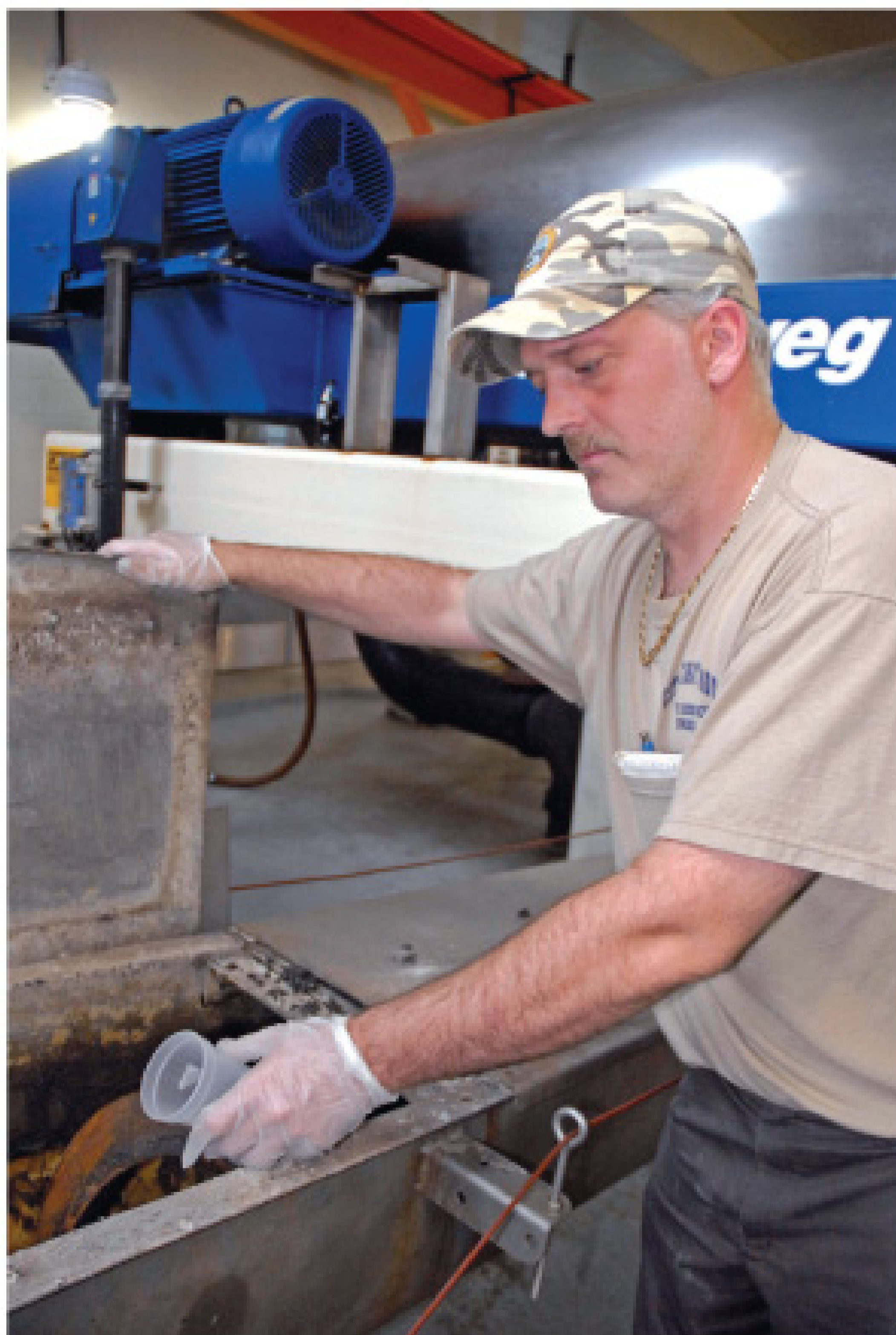
Operator Terry Davis with one of the plant's Flottweg high-G centrifuges.
