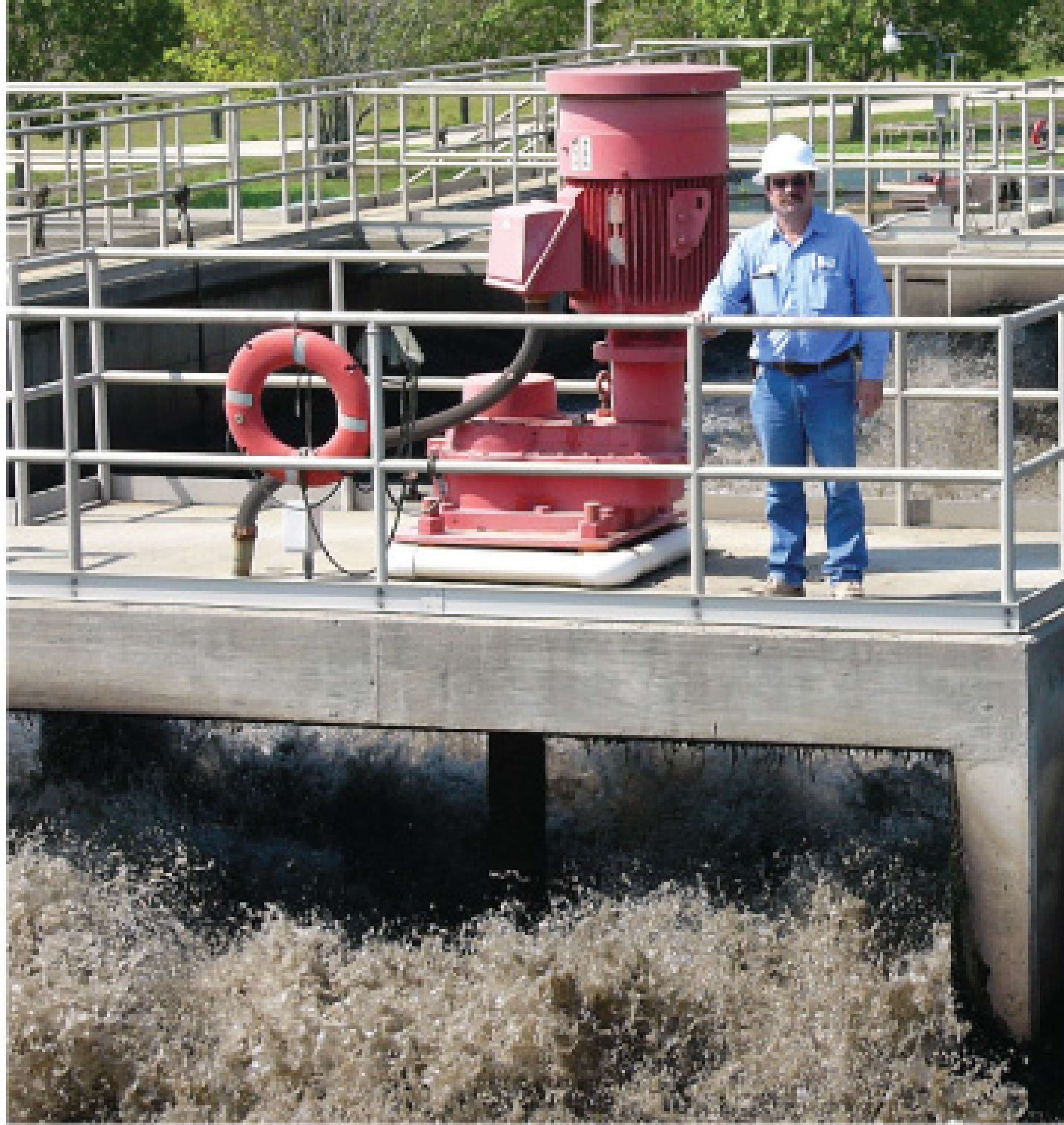
Chief operator Curtis Davis on an aeration basin.
