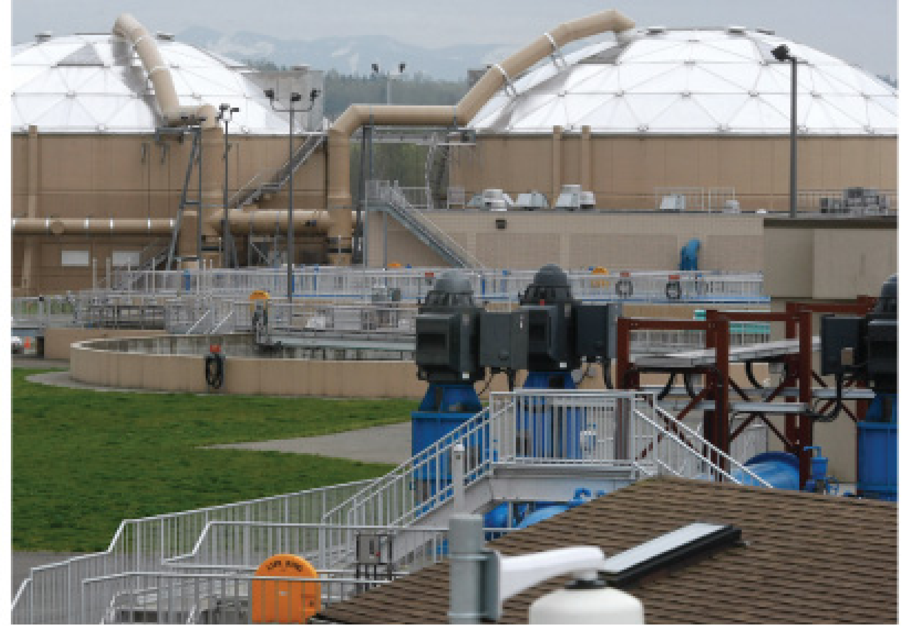
LEFT PHOTO: Water quality analyst Tim Rickman weighs wastewater solids collected on clarifier filters to determine TSS at different stages of clarification. ABOVE: The view east from the primary clarifier shows the secondary clarifiers, in the foreground, and two trickling filters.
