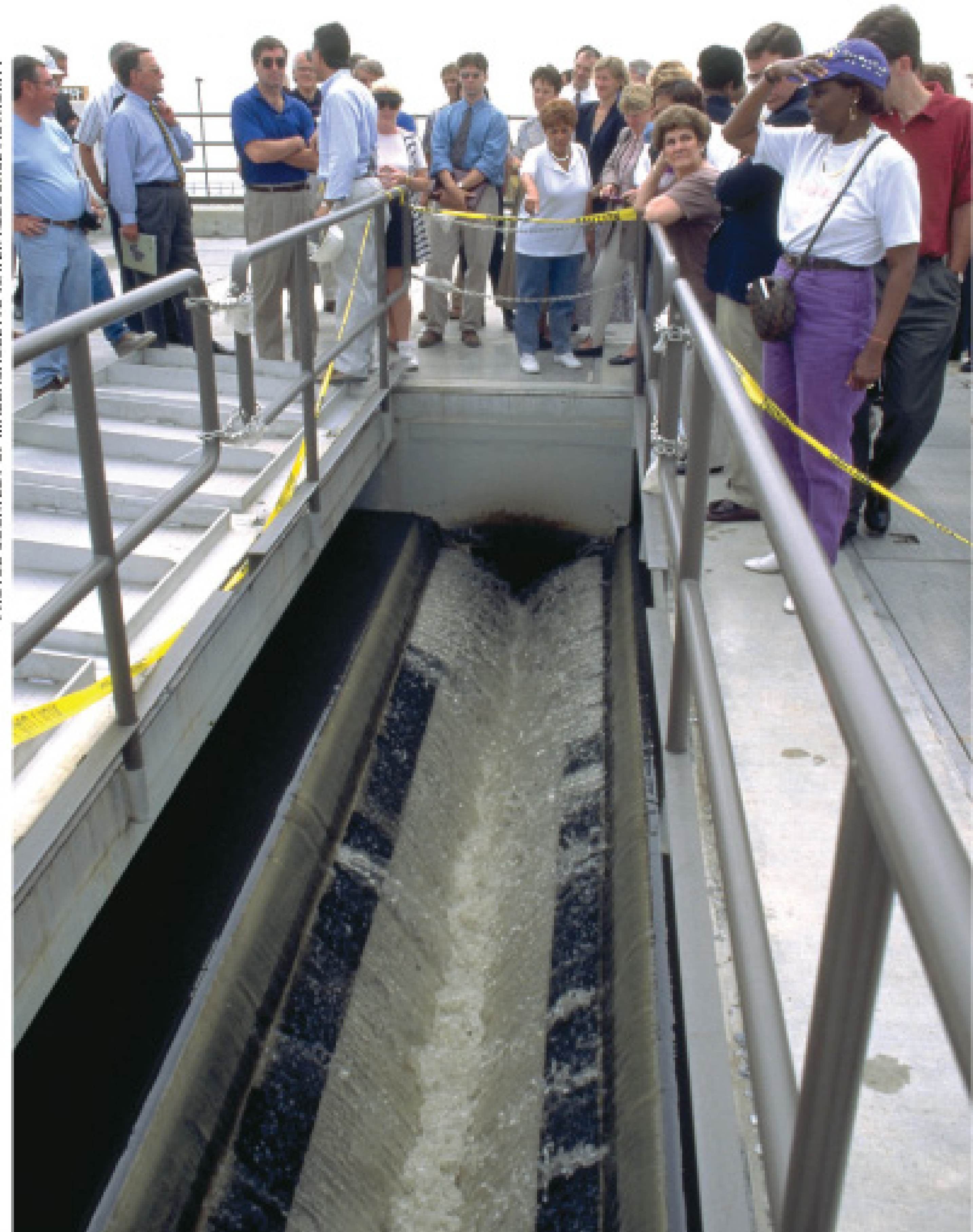
Since 1996, more than 50,000 visitors have toured the Deer Island Wastewater Treatment Plant including about 2,600 in 2008.
