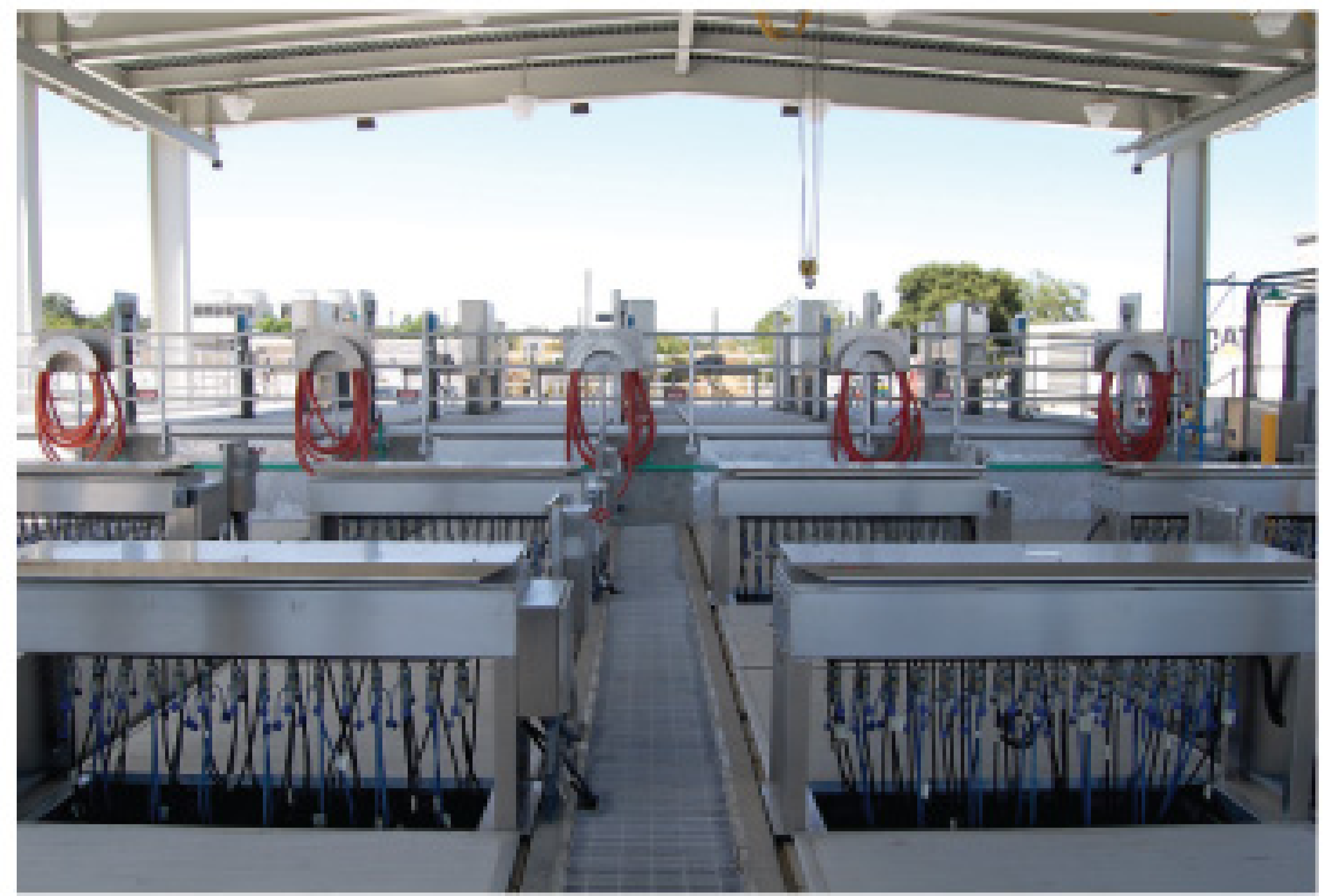
LEFT PHOTO: The 550-hp digester gas-fueled Dresser Waukesha engine at the Dry Creek Wastewater Treatment Plant in Roseville, Calif. ABOVE: The plant's five effluent channels are treated with a Trojan UV3000 Plus ultraviolet disinfection system. For each channel, there are four banks of 120 low-pressure, high-intensity lamps.
