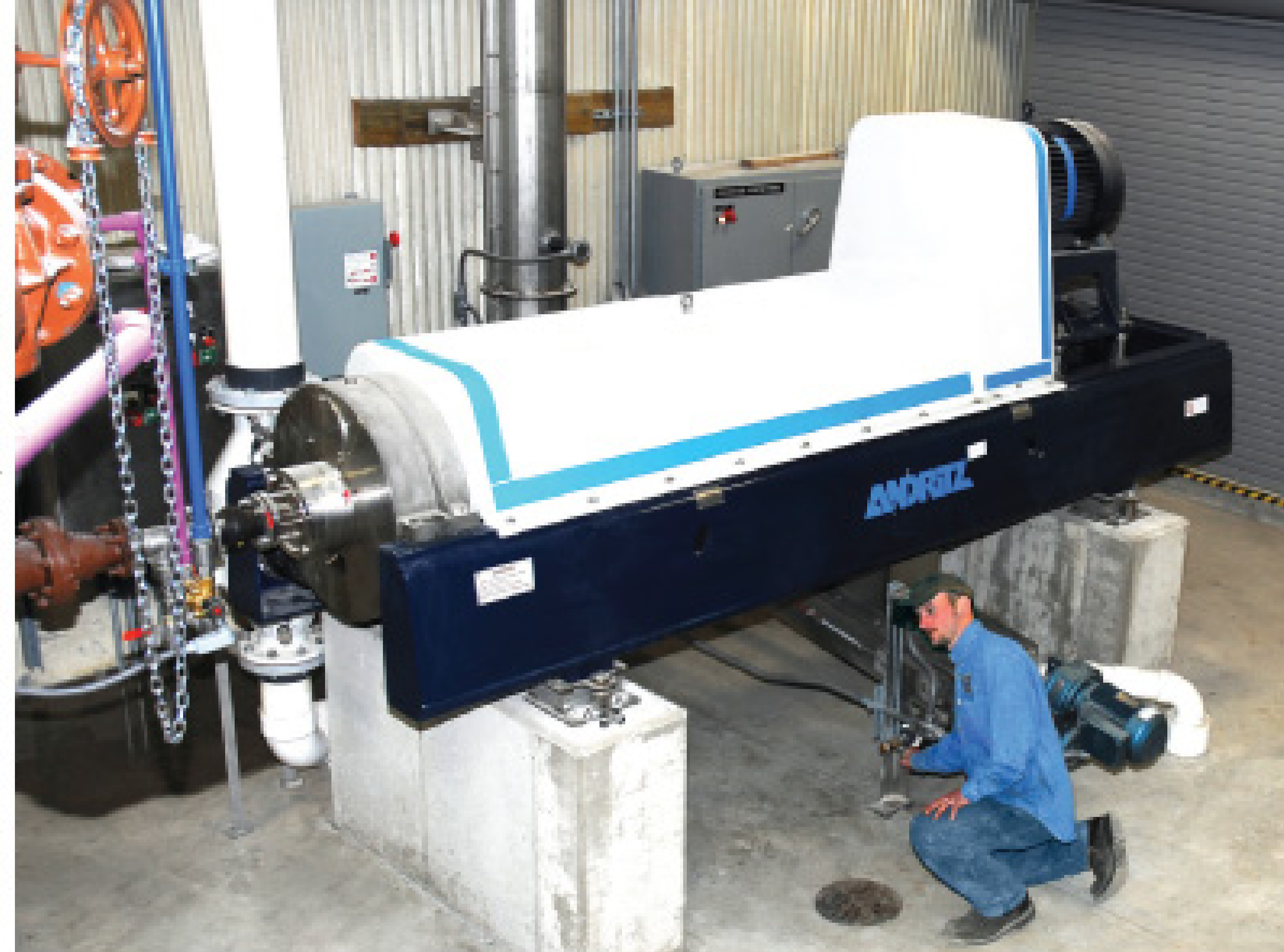
Class 4 operator Joe Cortese inspects an Andritz centrifuge at Lockport's newest wastewater treatment plant.
