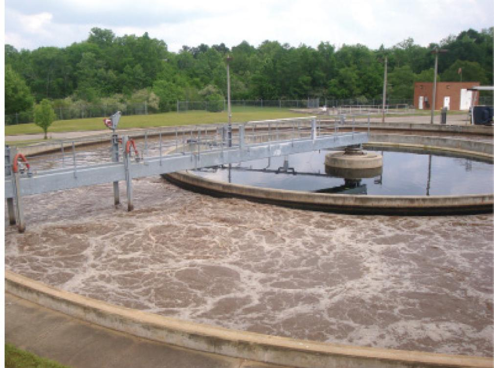
One of the two aeration basins at the Greenville Wastewater Treatment Plant that uses the Schreiber CSR process with a Hach SOLITAX sc suspended-solids analyzer and Hach Luminescent DO (LDO) probe.
