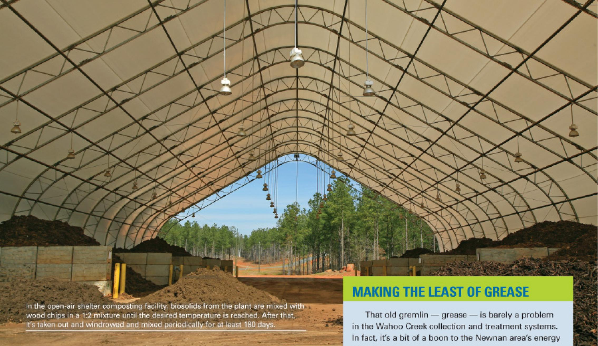
In the open-air shelter composting facility, biosolids from the plant are mixed with wood chips in a 1:2 mixture until the desired temperature is reached. After that, it's taken out and windrowed and mixed periodically for at least 180 days.
