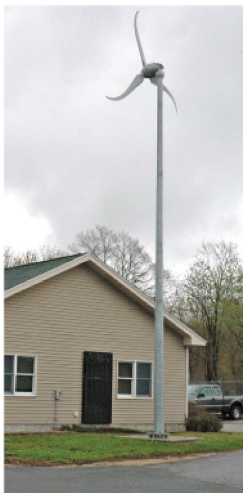
A 1.8-kW Skystream wind turbine supplements electric power for the plant’s administration building. A solar panel is on the side of the building.
