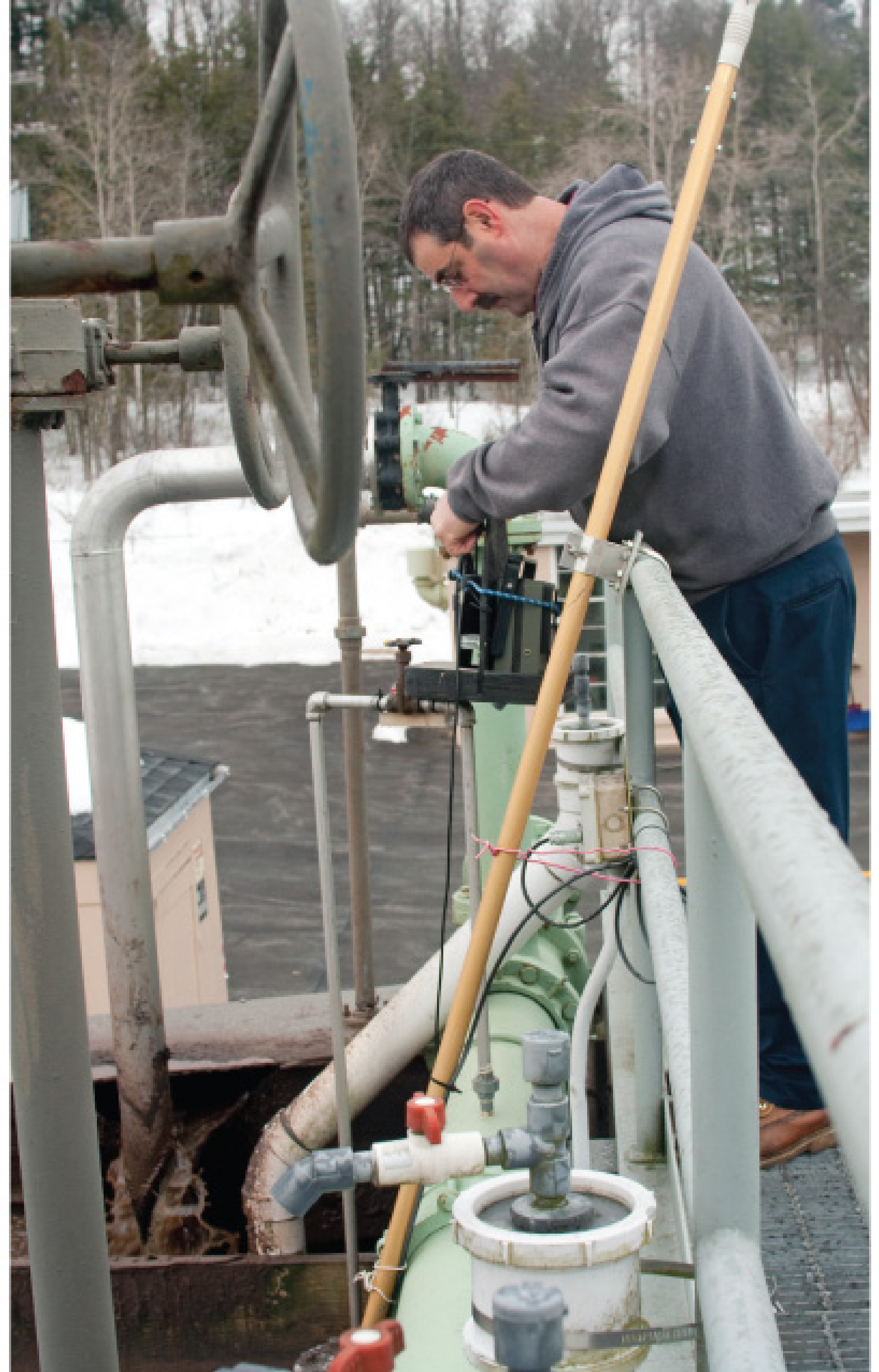
Langone checks the aeration tank with a YSI model 54A portable oxygen meter.
