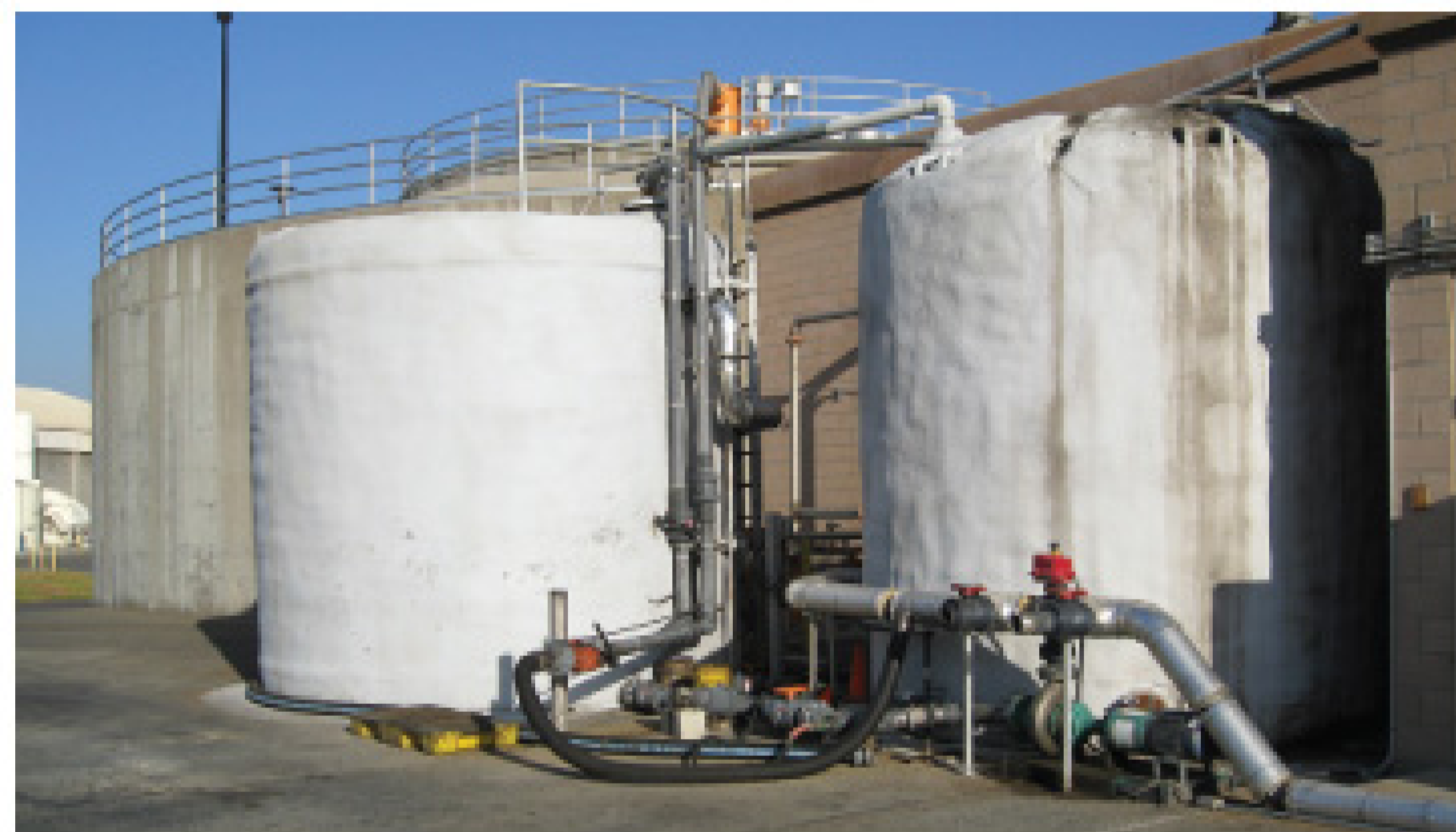
Two 10,000-gallon holding tanks store grease that will be fed into the digesters to increase methane production. Grease delivery trucks hook up here and pump the grease into the tanks, where it is circulated before being sent to the digesters.
