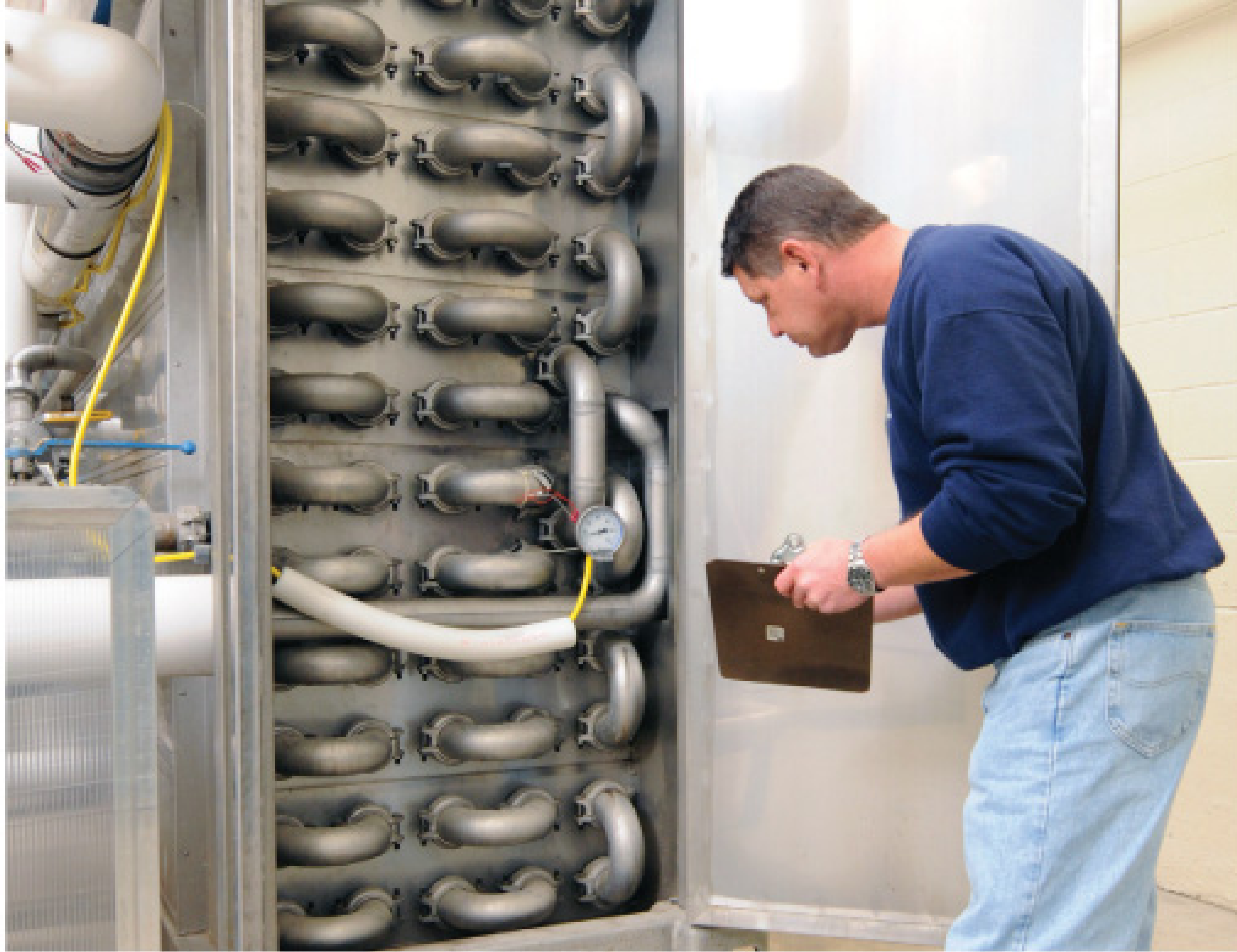
ABOVE: Jordan Kleinsmith takes readings from gauges that monitor the BioPasteur process heat exchanger. LEFT: A pig from Pipeline Pigging Products is used to scour heat exchanger lines. RIGHT: The BioPasteur system uses three 3,300-gallon tanks that operate in a sequential batch mode.
