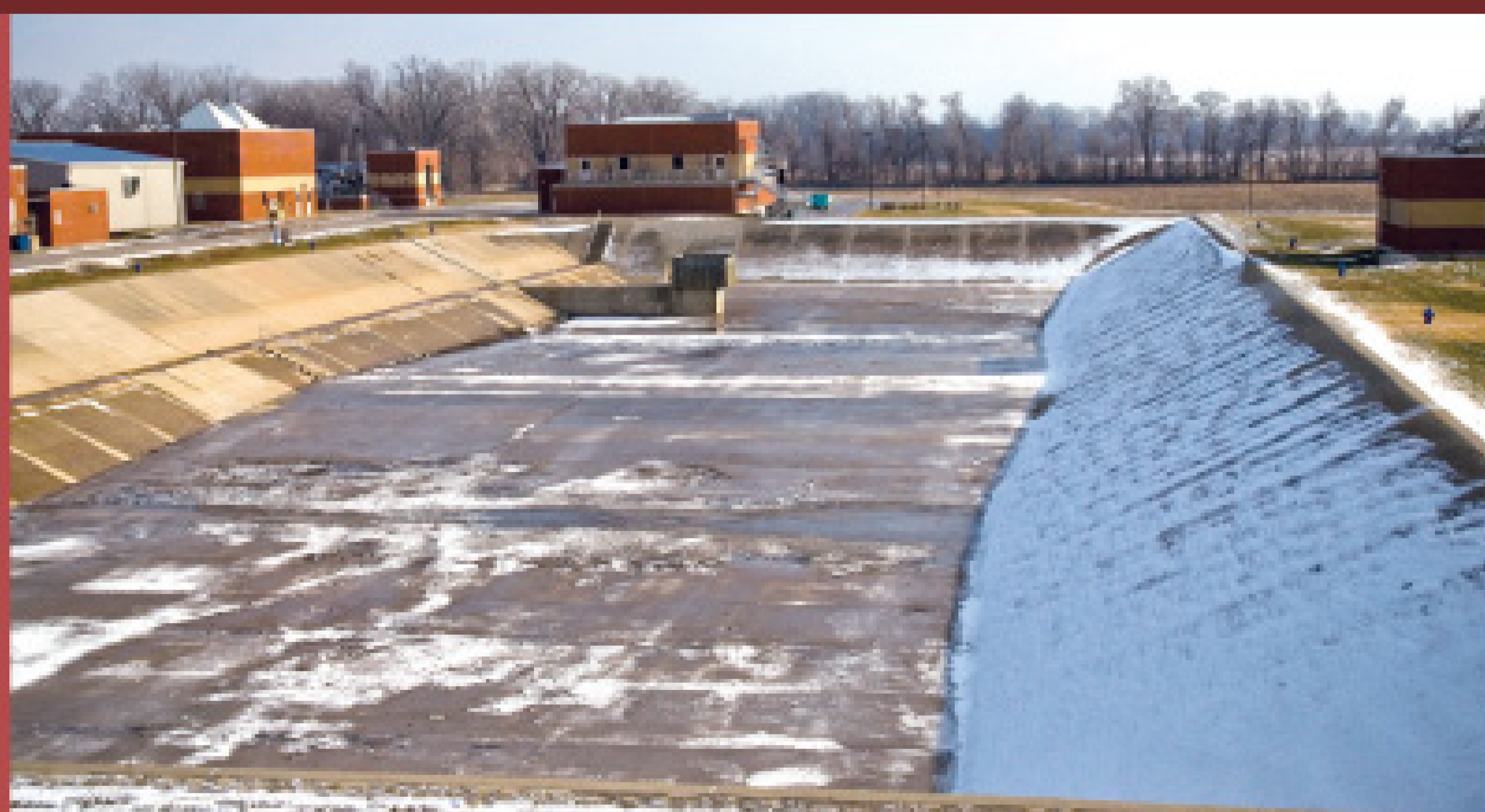
The excess flow storage basin is pictured with most of the plant's new buildings as of 2003. At the far end of the basin is the fine screen building. At left are the ACTIFLO process chemical storage buildings and the ACTIFLO treatment train and pump buildings.
