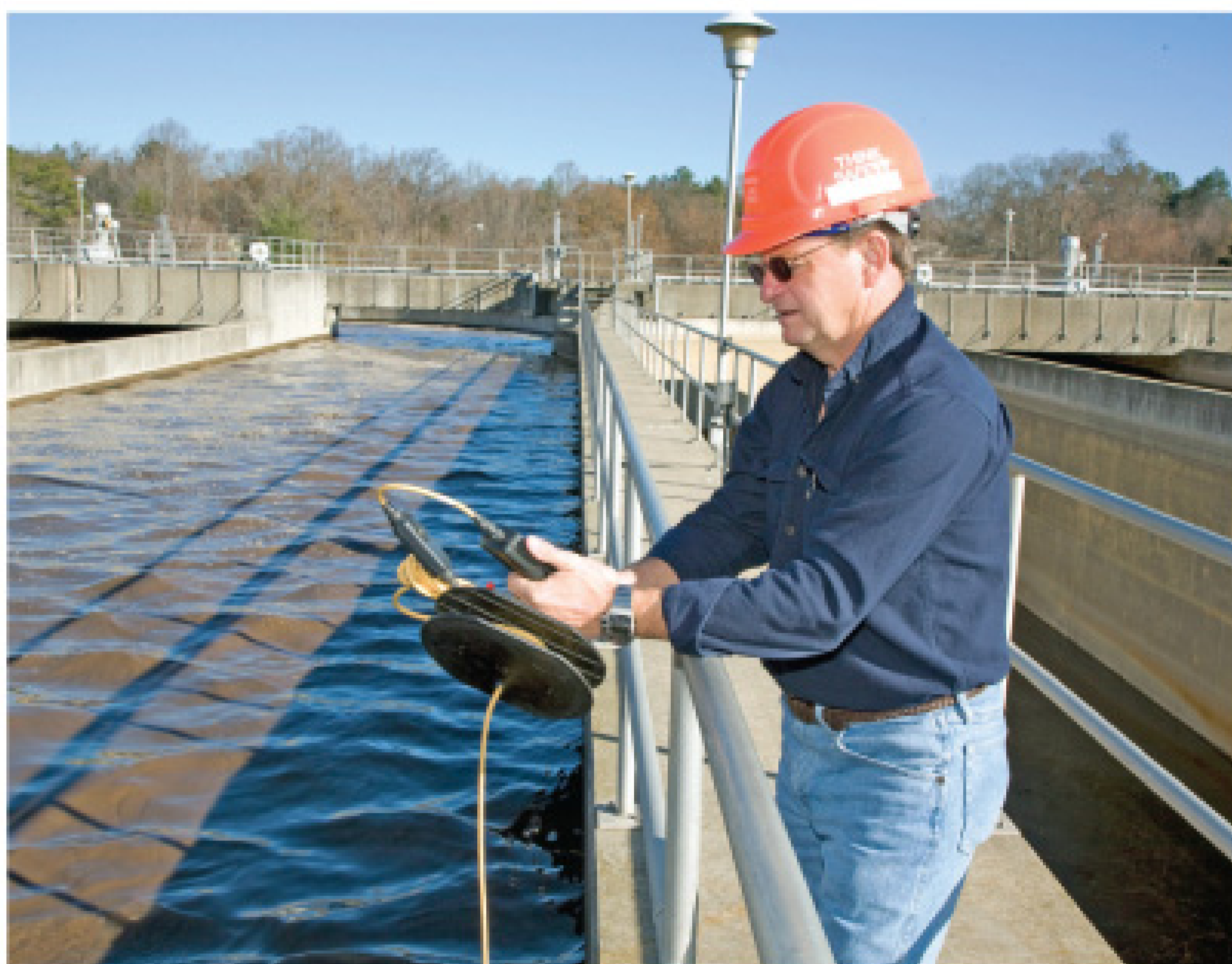
Tommy Smith, operator, takes dissolved oxygen measurements from the Carrousel oxidation ditch.
