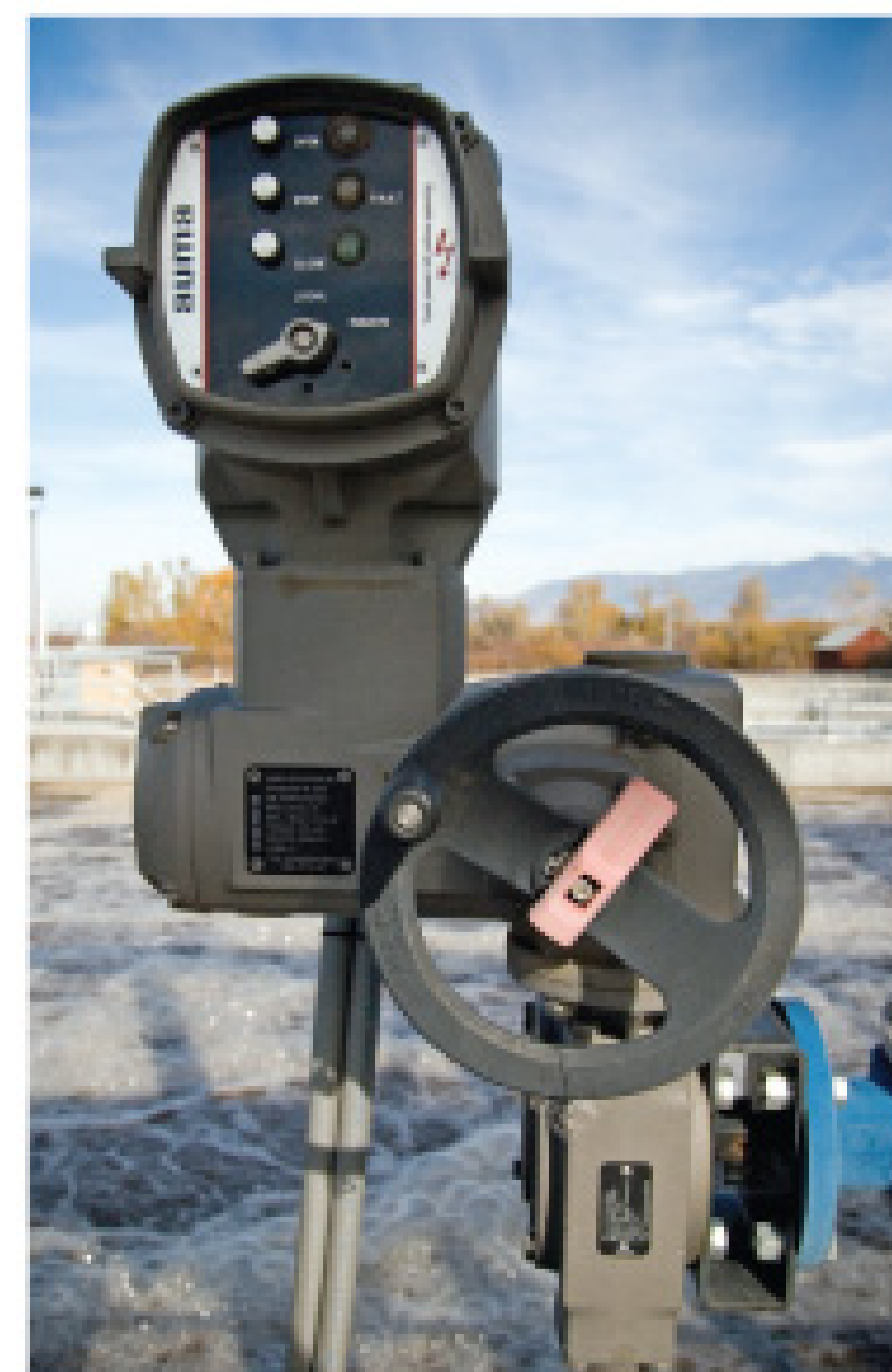
An aeration valve actuator from AUMA Actuators automatically opens and closes air valves to control the release of air into the aeration tanks.
