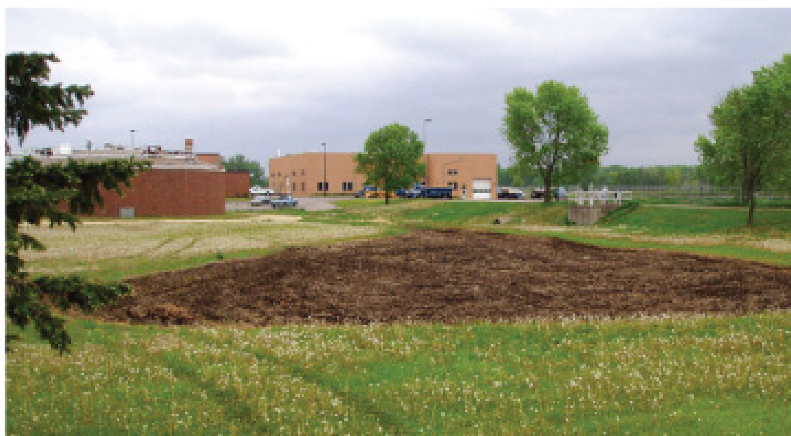
Three rain gardens allow stormwater to soak slowly into the rich loam, filtering out pollutants and reducing runoff. The gardens, ranging from 0.3 to 1.2 acres, are depressed basins planted with low-maintenance native grasses.
