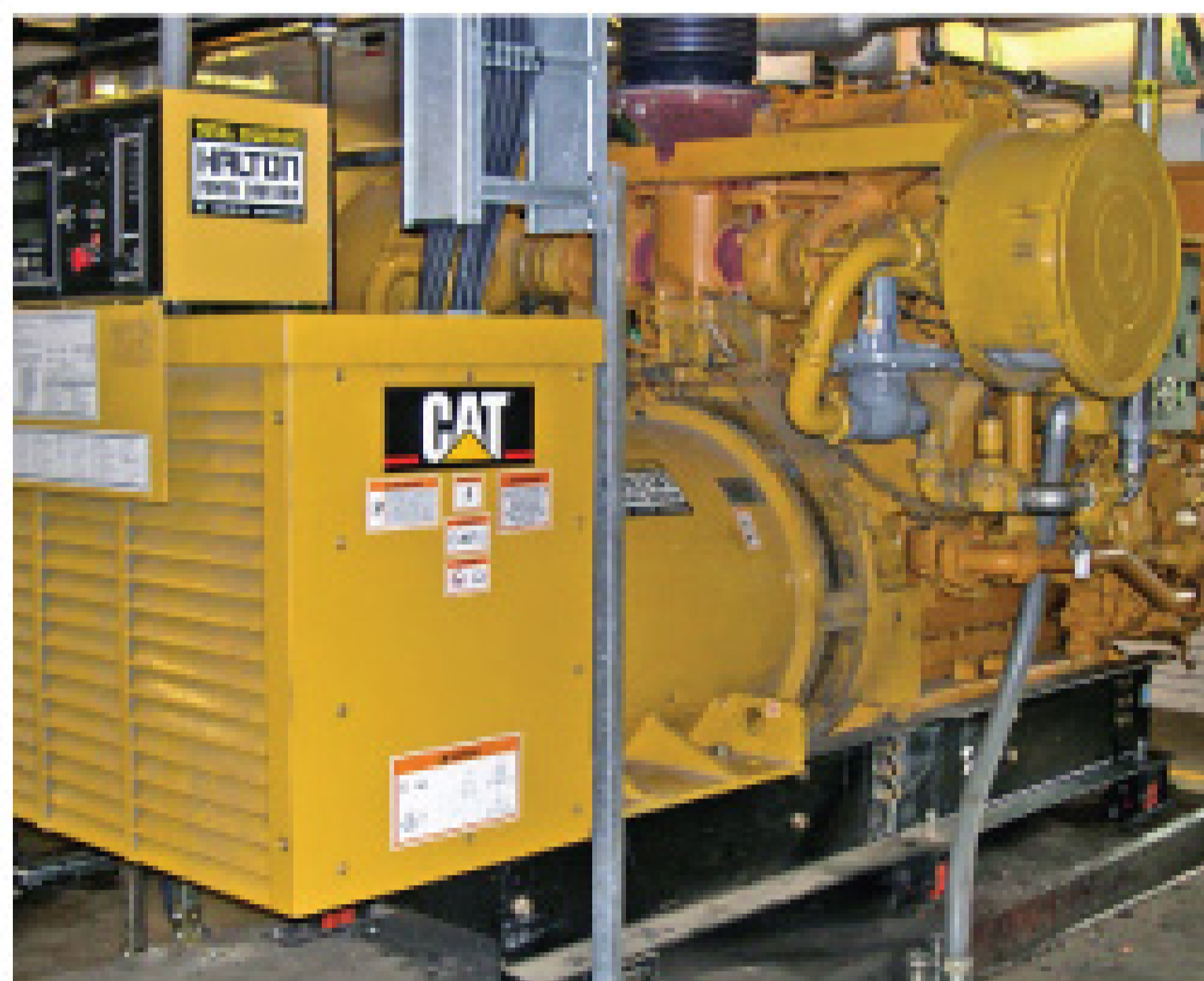
TOP PHOTO: Methane from the plant digesters is captured and treated for use in heating and power generation. LOWER LEFT: A 395-kW CAT combined heat and power system supplies nearly half of the plant's 800 kW peak load. Piping for the combined heat and power system.
