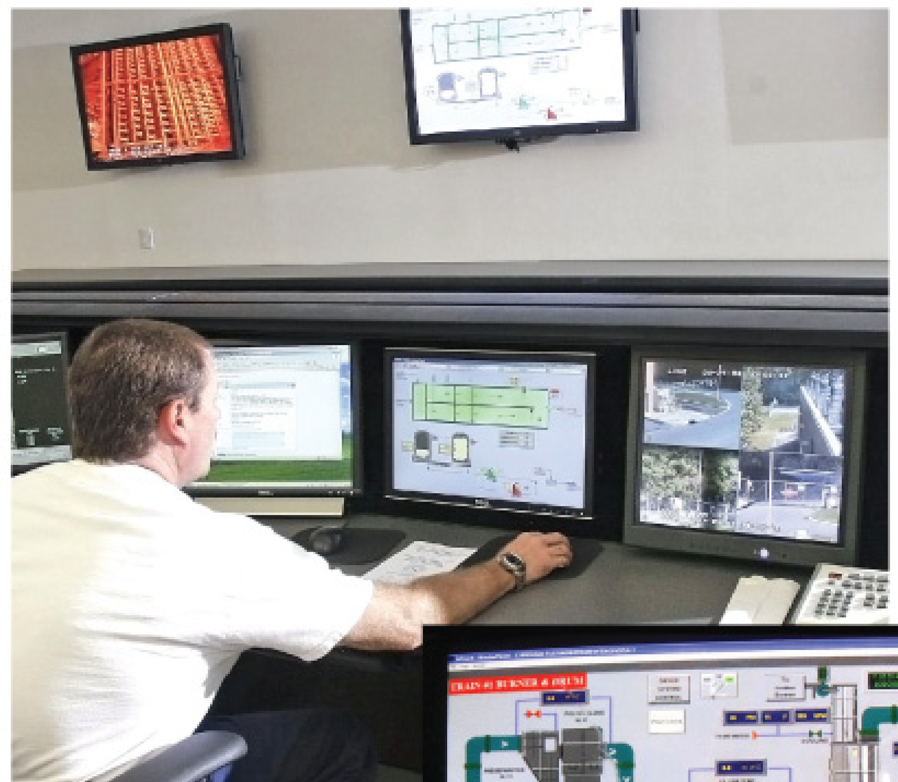
Above, a computer monitor display shows a schematic of the process for making OCEANGRO fertilizer at the Ocean County Utilities Authority. Operators can control the process from the computer. At right, a close-up of the process diagram.
