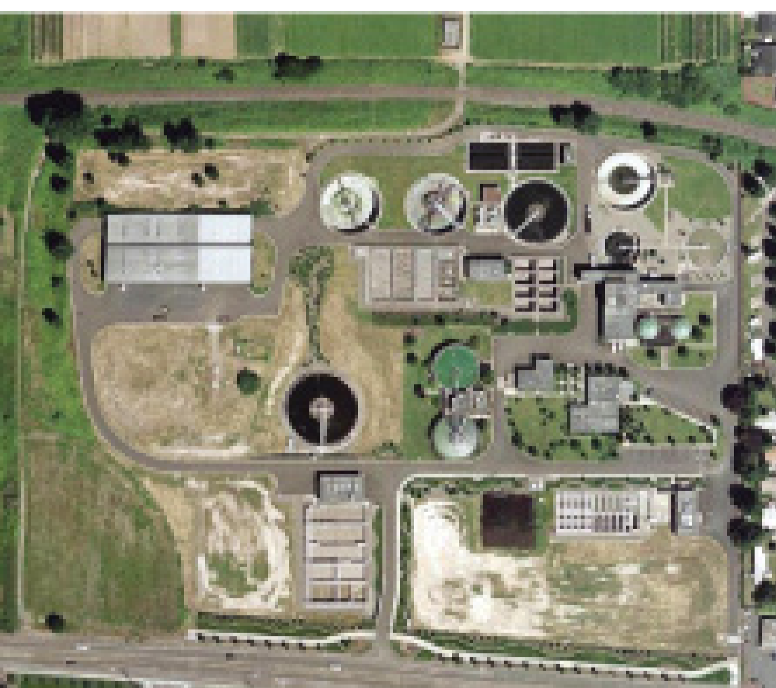
The current configuration of the Gresham Wastewater Treatment Plant. Solar panels are planned for the area shown in bottom right corner of the picture.
