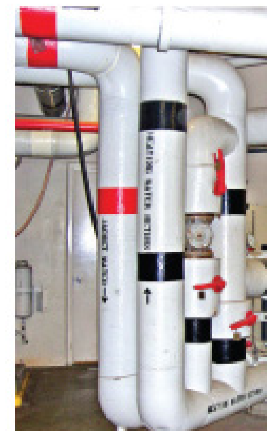
TOP PHOTO: Methane from the plant digesters is captured and treated for use in heating and power generation. LOWER LEFT: A 395-kW CAT combined heat and power system supplies nearly half of the plant's 800 kW peak load. Piping for the combined heat and power system.
